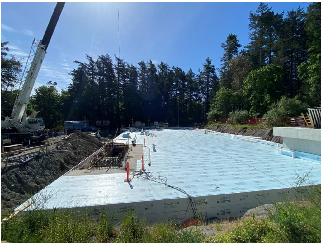
Figure 14 – Arbutus Attenuation Tank (Construction in progress)
