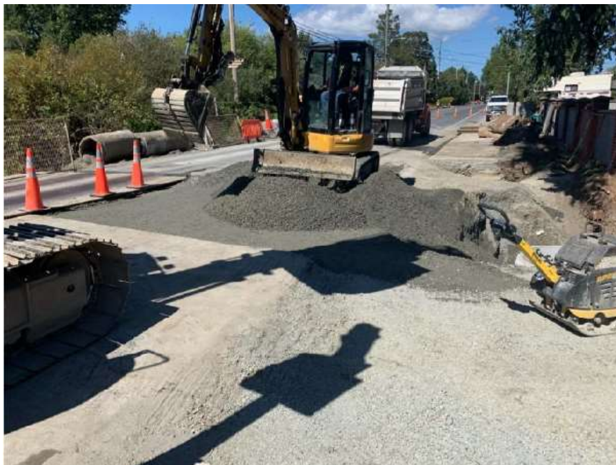
Figure 16– Residual Solids Pipes- Peers Creek – Base gravel being placed and graded over culverts.
