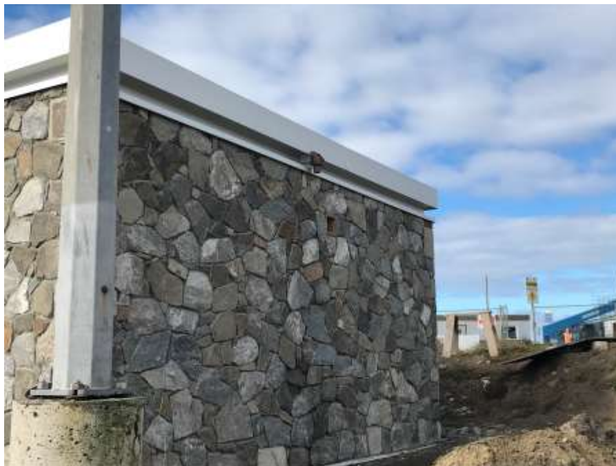
Figure 9–Clover Point Pump Station- Stonework masonry completed on exterior of public washroom.
