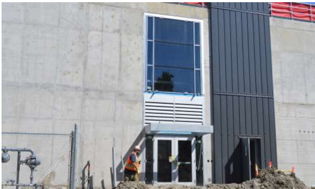
Figure 5- McLoughlin Point Wastewater Treatment Plant- Louvers installed at west entrance above doorway.
