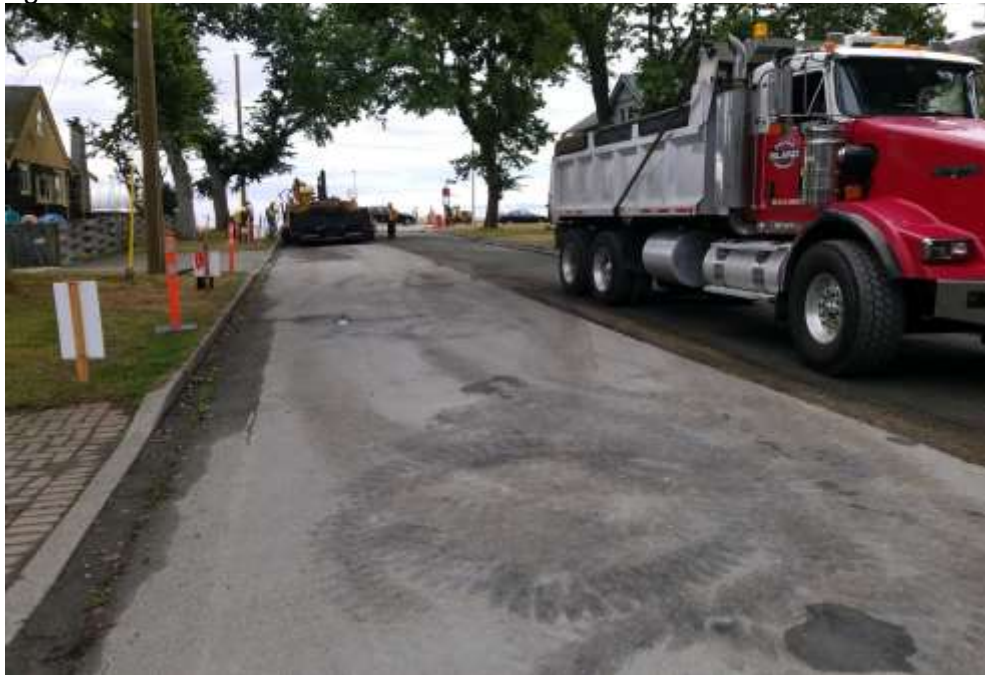
Figure 22–Trent Forcemain- base course paving on Eberts Street.
