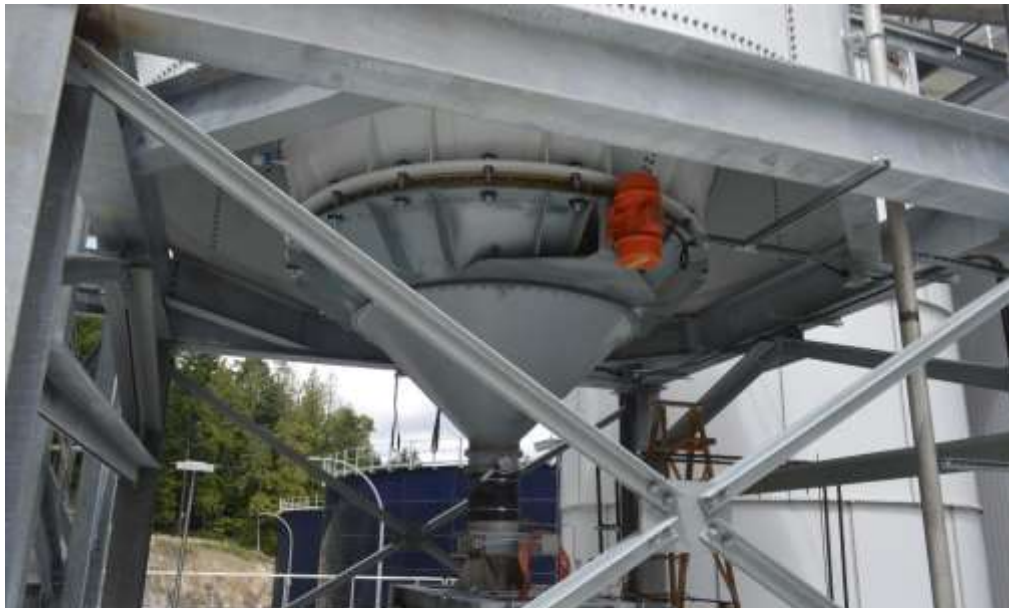
Figure 6– Residuals Treatment Facility- Product silo load out hopper.
