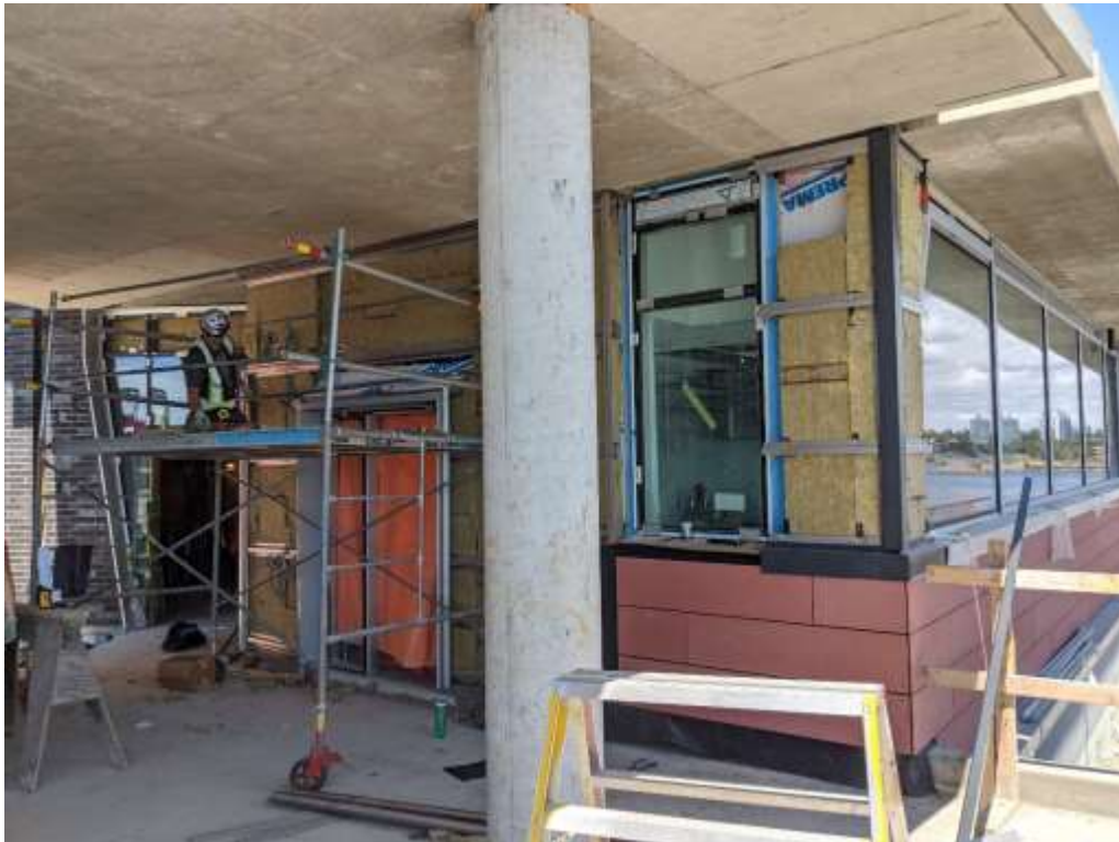
Figure 5– McLoughlin Point Wastewater Treatment Plant- Operations & Maintenance building level 1, south entrance façade insulation.
