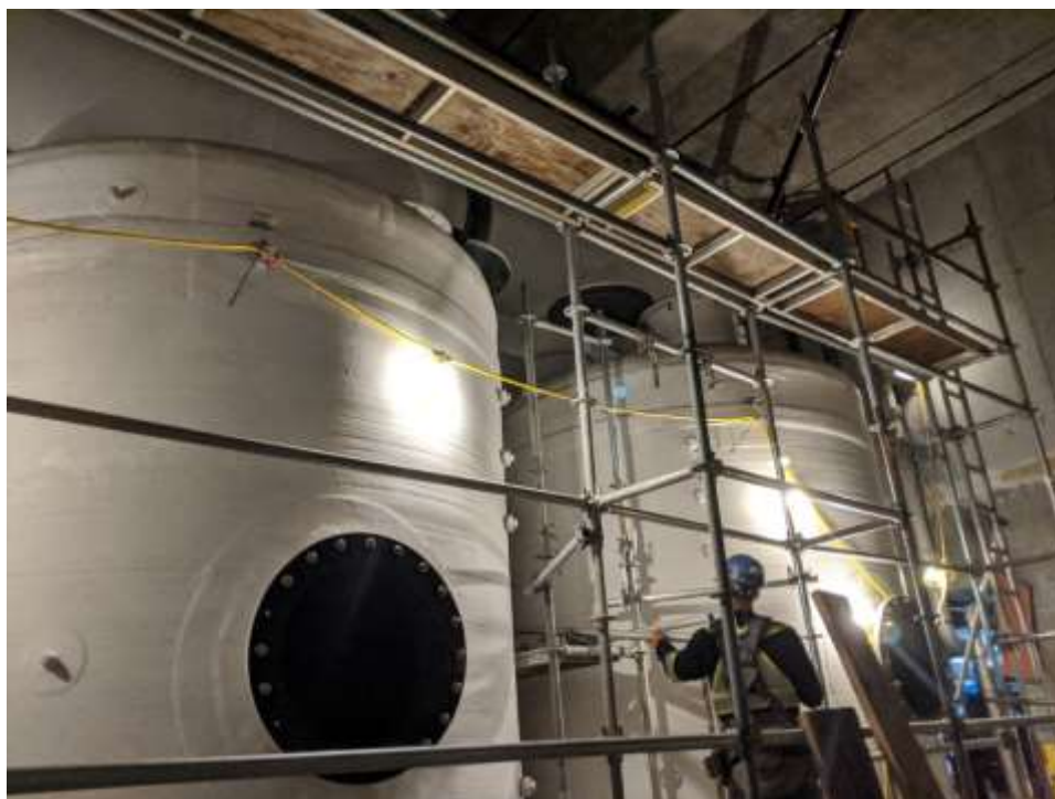
Figure 3– McLoughlin Point Wastewater Treatment Plant- Dirty Backwash Room, primary odour control carbon filter preparing to load media.
