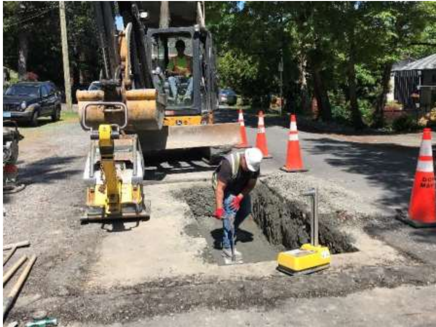
Figure 17-Residual Solids Pipes- Back fill and compaction on Grange Road after coupler repair.
