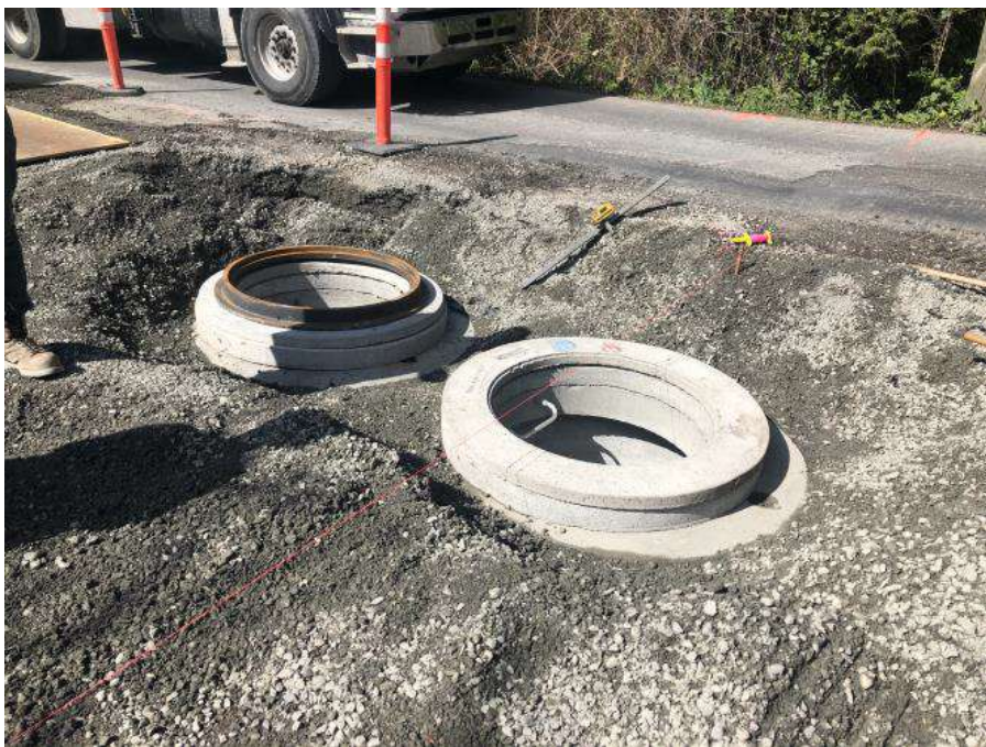
Figure 19-Residual Solids Pipes- Setting of grade rings at low point drain on Interurban Road.
