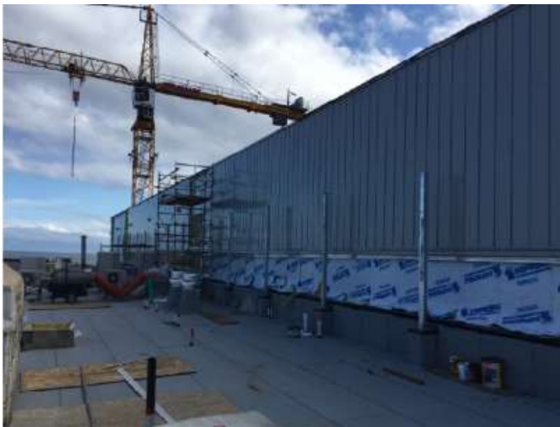
Figure 6– McLoughlin Point Wastewater Treatment Plant- Installing aluminium cladding on east face of Heat Recovery Room.
