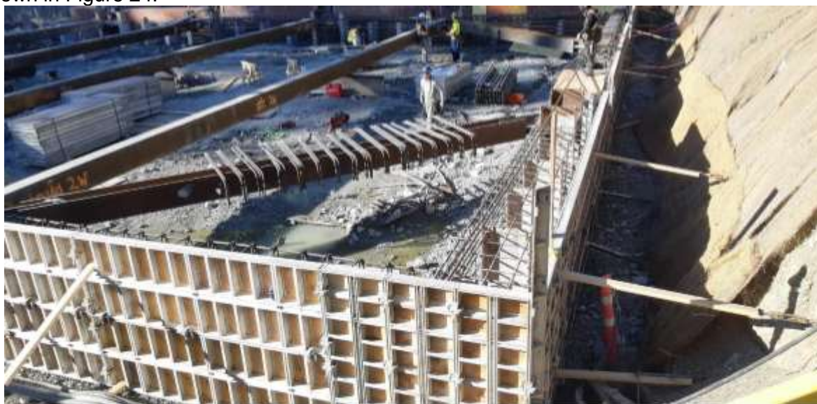
Figure 24–Arbutus Attenuation Tank–Installed diagonal and lateral struts atop the secant piles, formwork and rebar installed for section 1 of ring beam.
