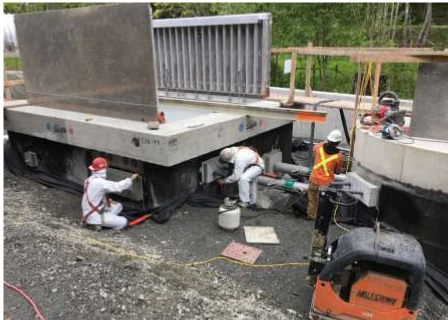
Figure 22–Residual Solids Pump Stations– Pump Station 1 – Grouting and sealing of pipe penetrations in valve chamber.
