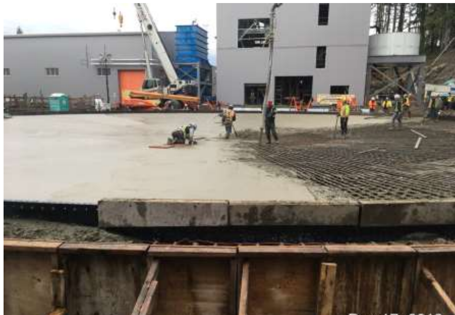
Figure 7– Residuals Treatment Facility- Concrete placement for digester #3 tank slab.
