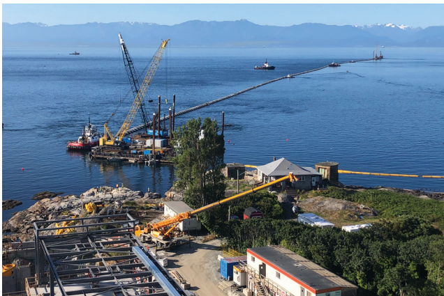
The outfall pipe being installed in July is 2.25m in diameter and 1.92km long.
