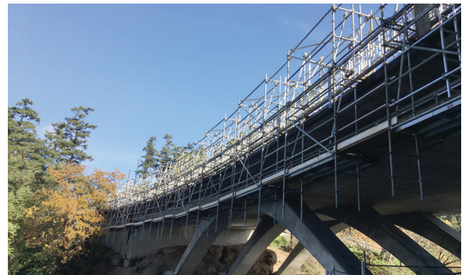
Scaffolding on the Tillicum Bridge to install the RSCL pipe.
