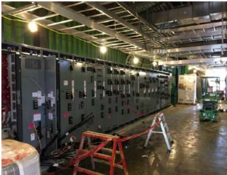
Figure 6– McLoughlin Point Wastewater Treatment Plant- Landing electrical feeds in Motor Control Centres.
