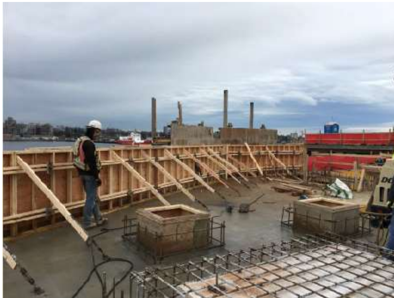
Figure 5– McLoughlin Point Wastewater Treatment Plant-Forming odour control roof parapet and roof penetration curbs.
