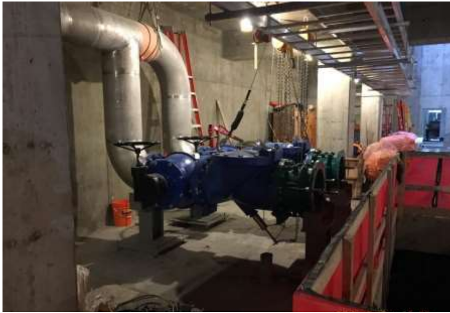
Figure 4– McLoughlin Point Wastewater Treatment Plant- Installation of control valves and check valves for backwash piping.
