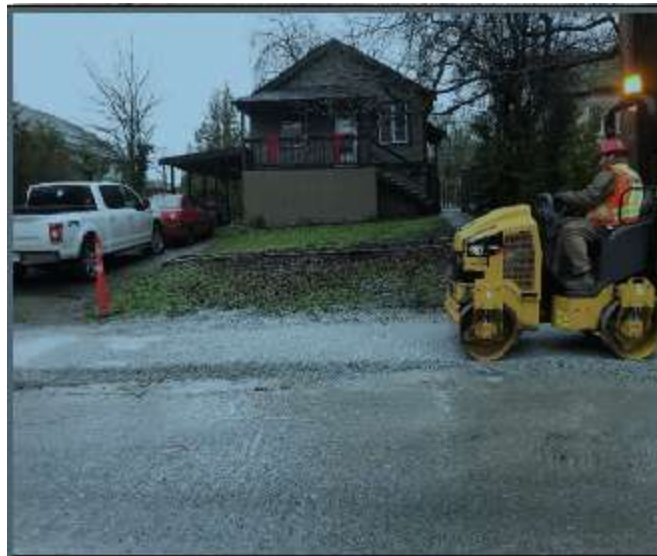
Figure 22–Residual Solids Pipes- Compacting gravel on Vincent Ave.
