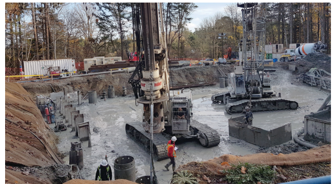
Concrete caisson piles are being installed at the site of the Arbutus Attenuation Tank.
