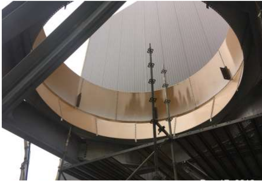
Figure 8– Residuals Treatment Facility- Product storage silo being constructed on south side of dryer building.
