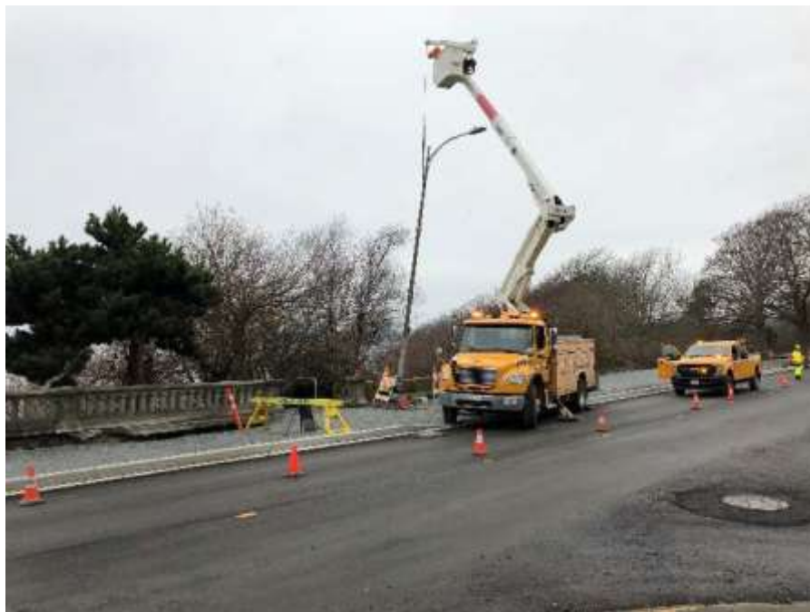
Figure 19–Clover Forcemain– Lamp standard installation near Paddon Ave.
