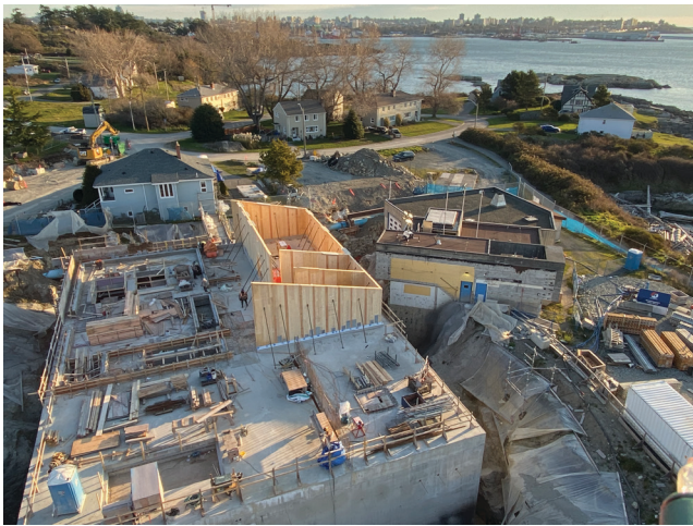
The above-ground timber structure is being constructed at Macaulay Point Pump Station.
