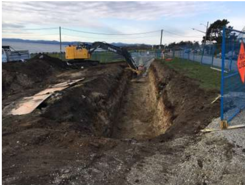
Figure 11–Clover Point Pump Station- Excavation for forcemain installation.
