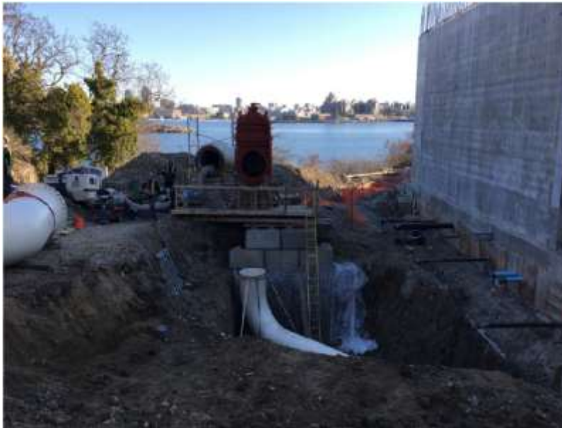
Figure 2– McLoughlin Point Wastewater Treatment Plant- Installation of pig receiver station, piping and valves.
