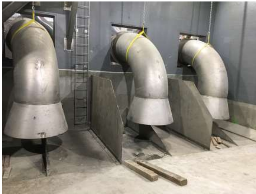
Figure 14- Clover Pump Station - Installation of suction spools.
