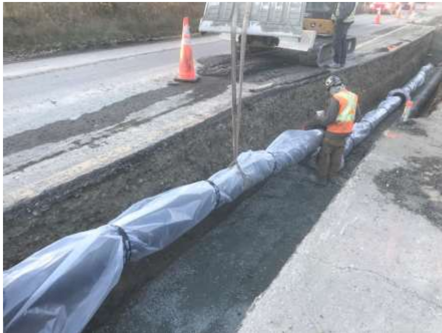
Figure 23–Residual Solids Conveyance Line- Ductile iron pipe installation on Interurban Rd near North Road.
