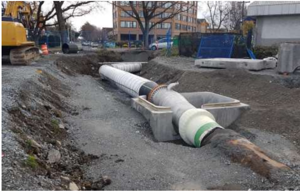
Figure 17–Clover Forcemain- Final tie-in to the Harbour Crossing pipe in the transition chamber.
