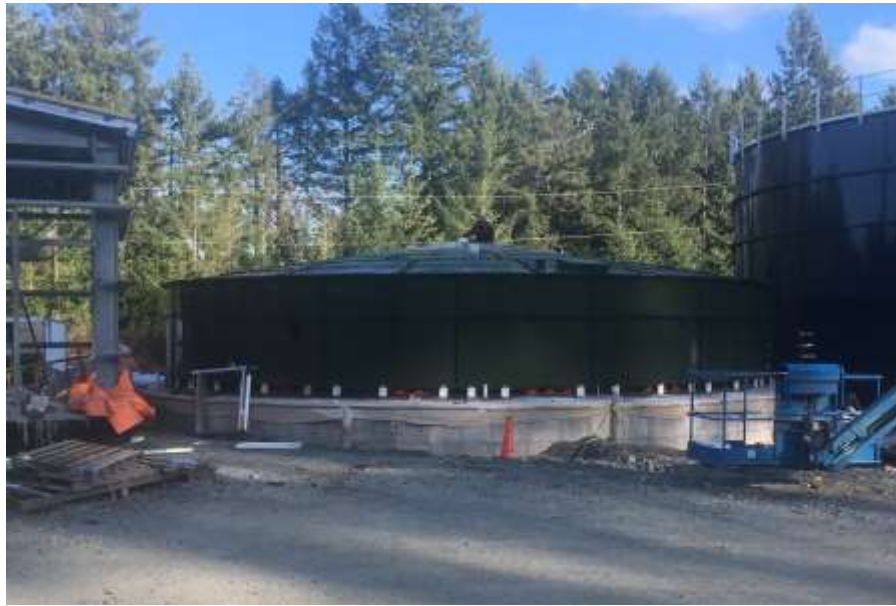
Figure 7– Residuals Treatment Facility- Installation of bolted steel roof panels on water storage tank.
