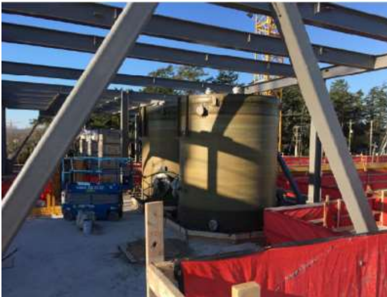
Figure 3– McLoughlin Point Wastewater Treatment Plant- Setting of Secondary Chemical Tanks.
