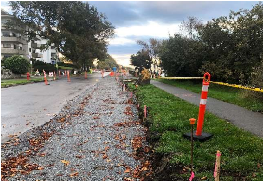
Figure 17–Clover Forcemain- Curb and gutter removals and base preparation along Dallas (South Side - Douglas to Government)
