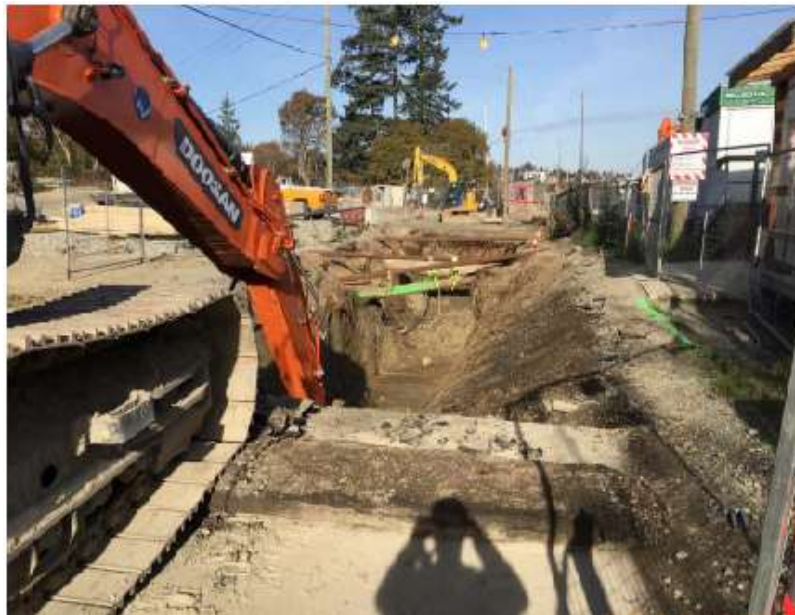
Figure 3– McLoughlin Point Wastewater Treatment Plant- Excavation of Macaulay forcemain pipe trench on Victoria View Road
