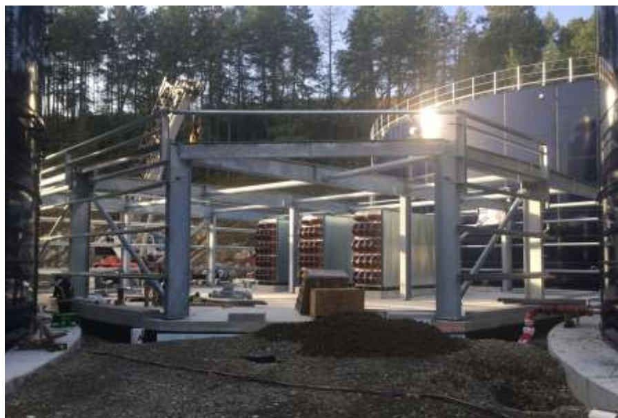
Figure 7– Residuals Treatment Facility- Installation of insulated metal cladding support members on Digester Equipment Building.
