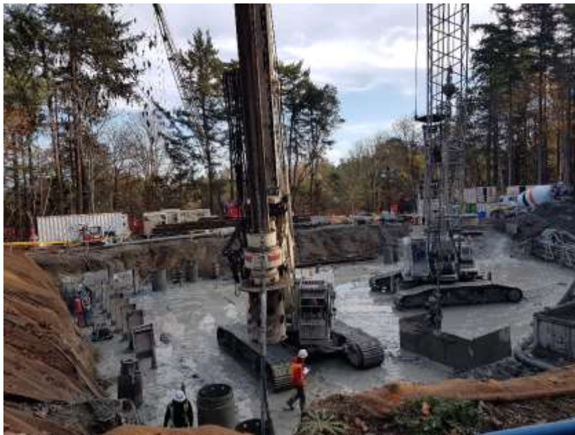
Figure 28–Arbutus Attenuation Tank- Installation of Secant Piles.
