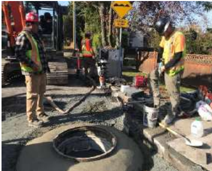
Figure 23-Residual Solids Conveyance Line- Placing concrete around manhole grade rings and frame on Selkirk Ave
