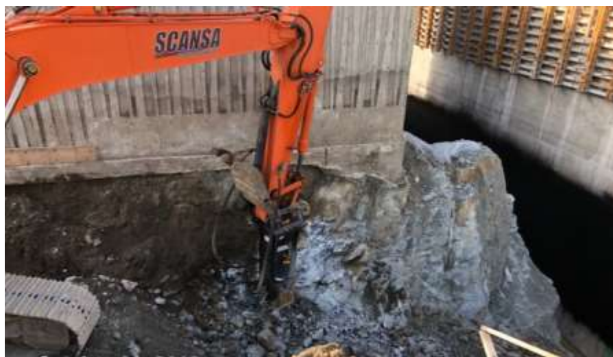
Figure 15–Macaulay Point Pump Station- Rock removal between diversion chamber and existing pump station.
