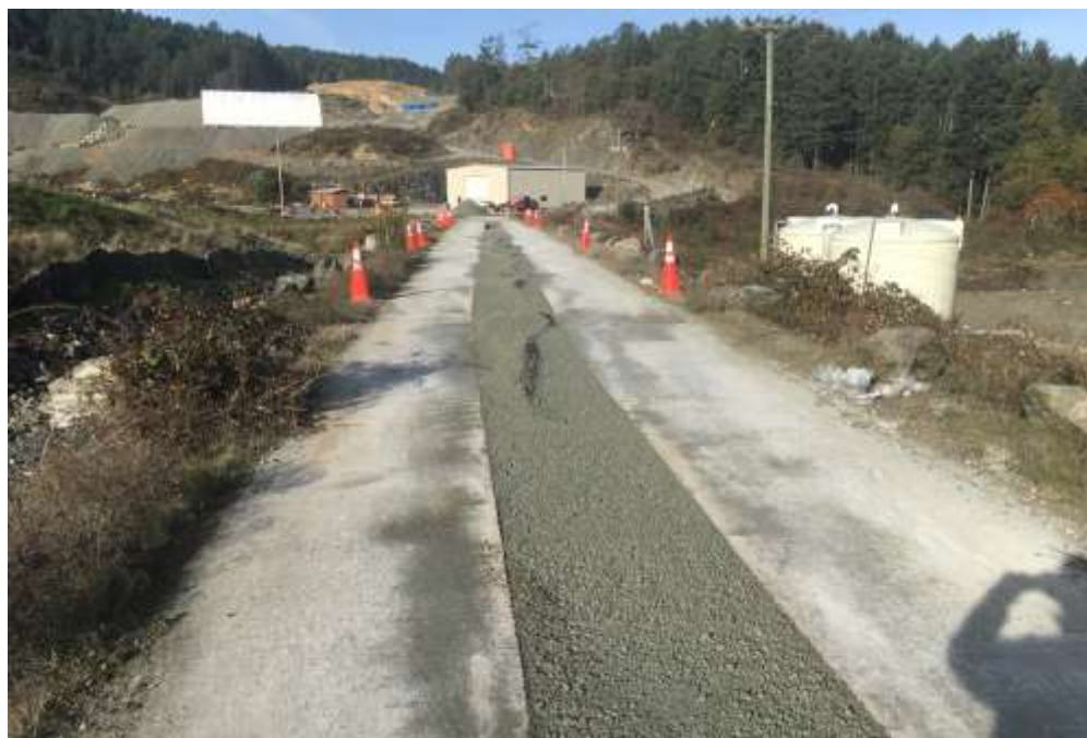
Figure 25–Residual Solids Pump Stations and Bridge Crossings – Watermain trench backfilled west of gas plant.
