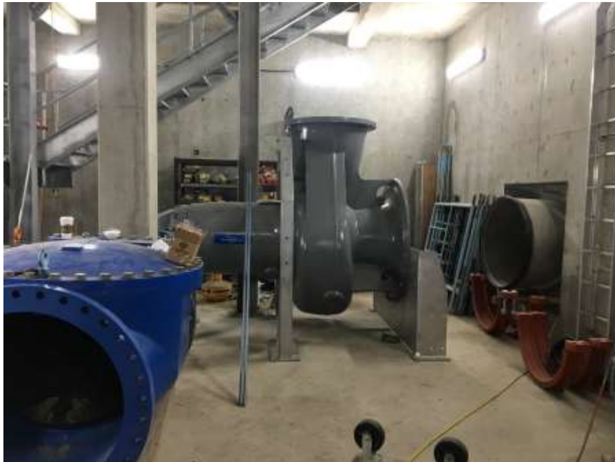
Figure 11–Clover Point Pump Station- Storm pump.
