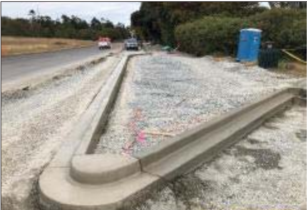
Figure 18–Clover Forcemain- Dallas Road curb and gutter installed
