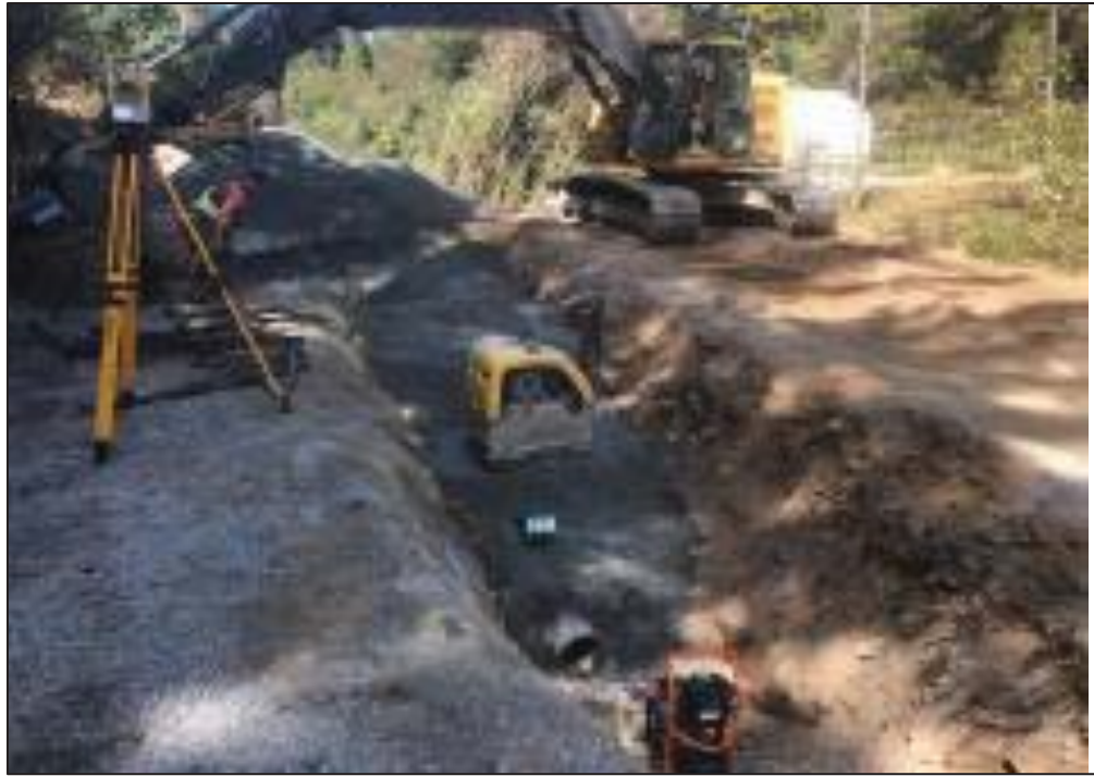
Figure 27–Residual Solids Pump Stations and Bridge Crossings – Backfilling the Residual Solids Forcemain at Pump Station 1 in lifts.
