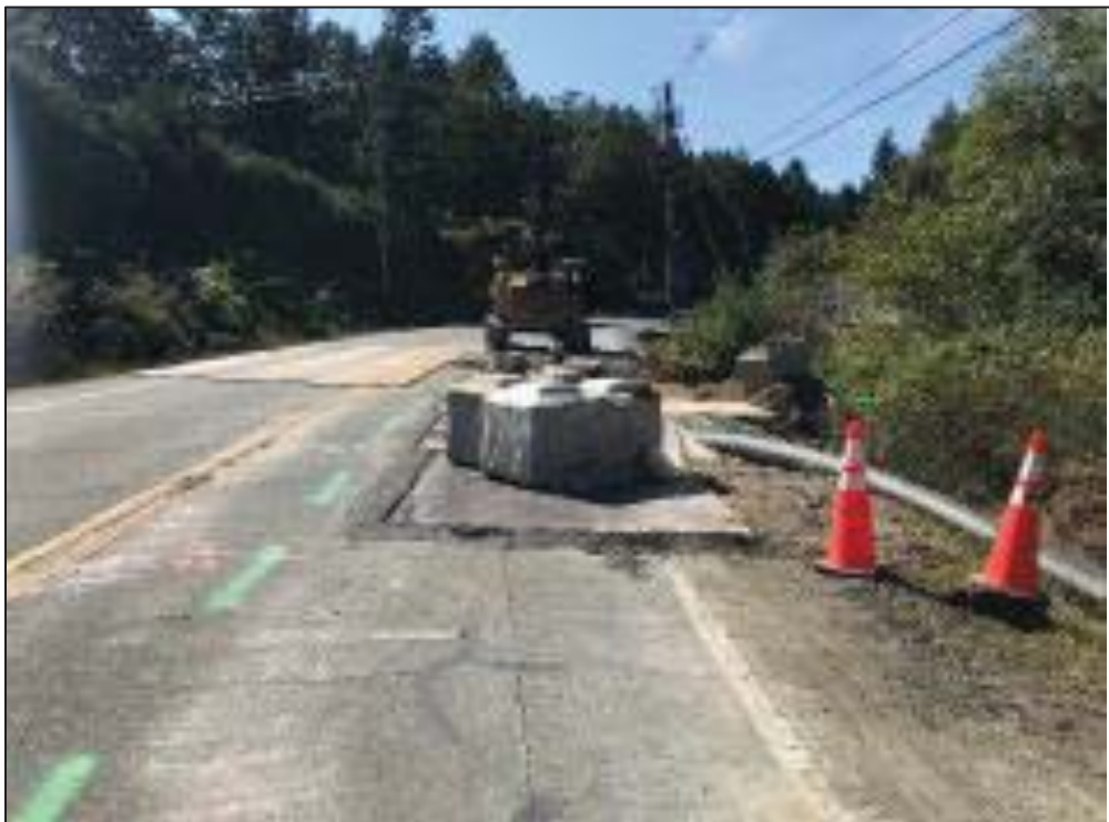
Figure 26 –Residual Solids Pump Stations and Bridge Crossings- Adjusting and stabilizing road plates on Willis Point Road
