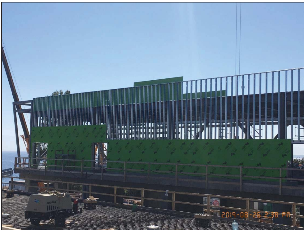
Figure 6- McLoughlin Point Wastewater Treatment Plant- Installing exterior sheathing for electrical room and room parapet.
