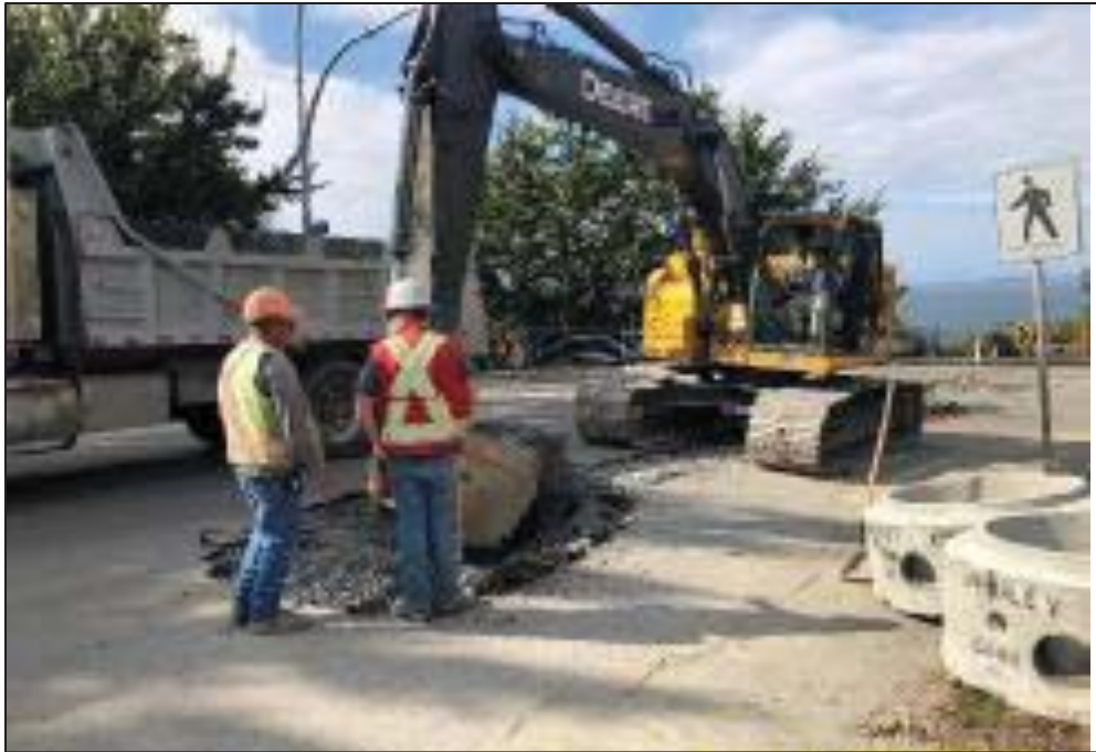
Figure 19—Clover Forcemain—commence excavation for City of Victoria sanitary main relocates.
