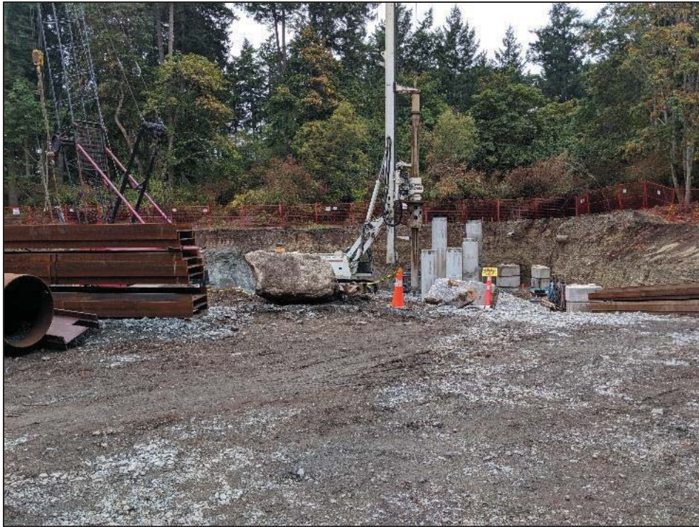
Figure 28–Arbutus Attenuation Tank- Drilling operation of Secant Pile
