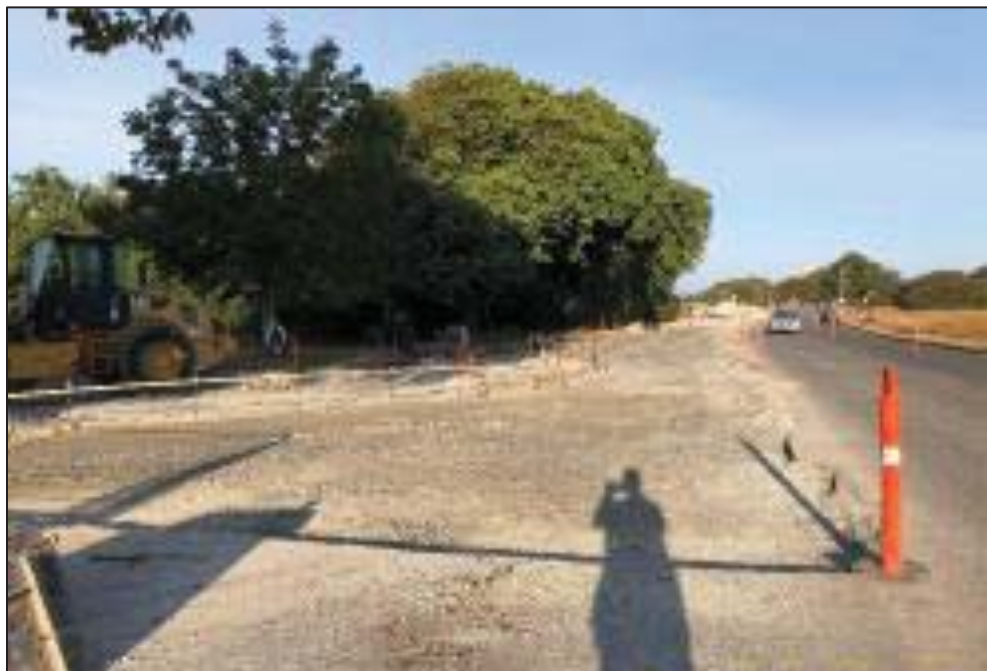
Figure 20—Clover Forcemain—Curb and gutter string set.
