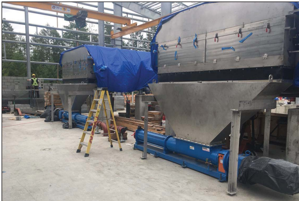
Figure 10– Residuals Treatment Facility- Installation of screw conveyors and mechanical piping for gravity belt thickeners.
