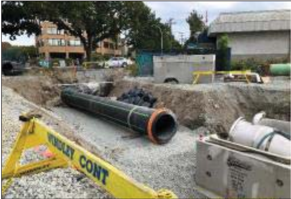
Figure 17–Clover Forcemain-Ogden Point - Weld-Neck Flange and transition chamber.
