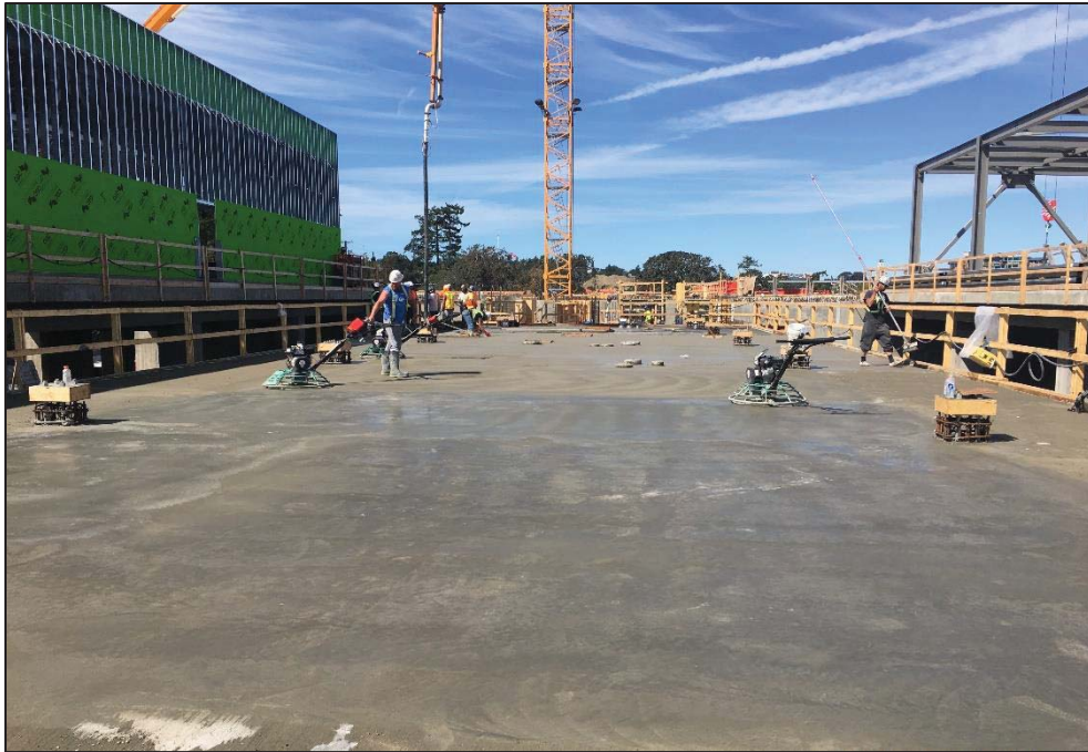
Figure 5- McLoughlin Point Wastewater Treatment Plant- Pouring and finishing BAF blower room slab.
