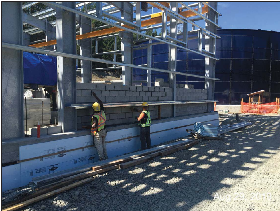
Figure 8- Residuals Treatment Facility- Masonry block wall construction ongoing in residuals handling building.
