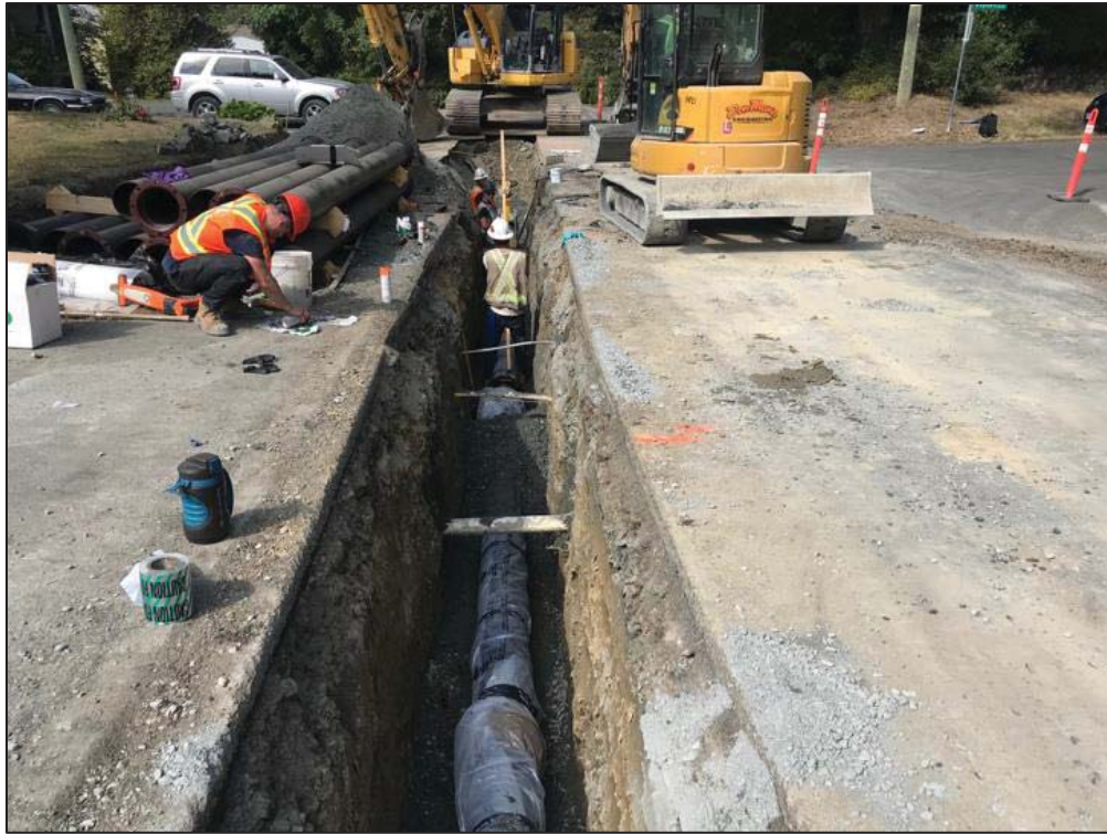
Figure 24–Residual Solids Conveyance Line- Ductile iron residual solids forcemain being installed in Segment 2, Grange Road between Violet Ave and Gardenia Court.
