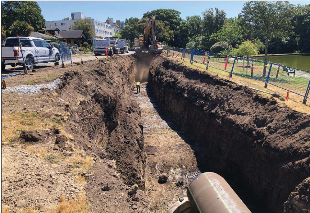
Figure 19–Clover Forcemain- Trenching advanced through Holland Point Park (Yacht Pond)
