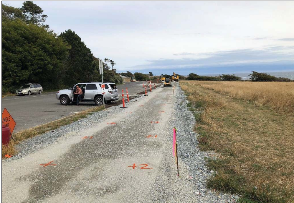
Figure 21–Clover Forcemain-Cycle Track Base Preparation (Clover Point).
