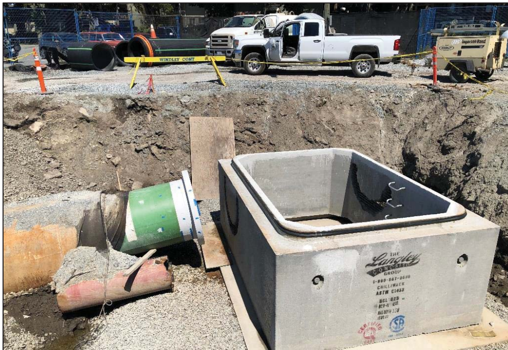
Figure 18–Clover Forcemain- Weld-Neck Flange welded and foundation and lower section of transition chamber installed.
