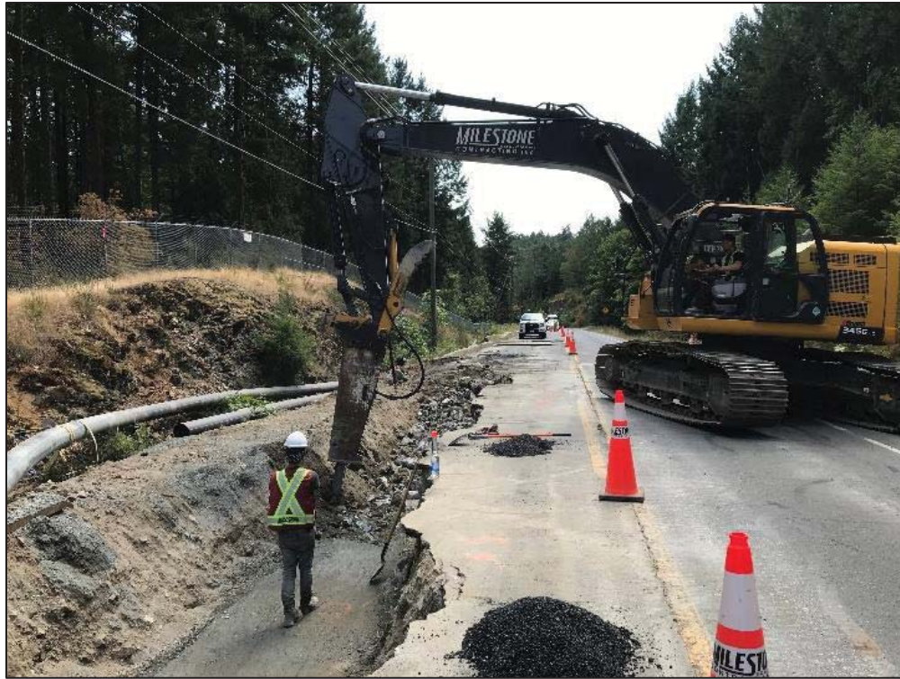
Figure 27 –Residual Solids Conveyance Line- Break rock in the trench at Willis Point Road
