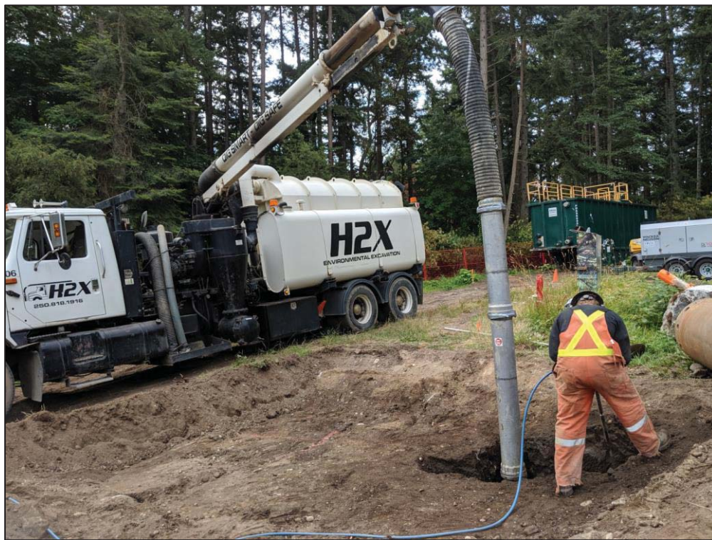
Figure 29–Arbutus Attenuation Tank- Daylighting existing utilities
