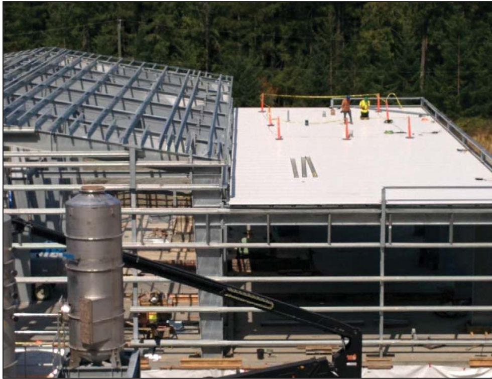
Figure 8- Residuals Treatment Facility- Residual Handling Building structural steel installation: roof bracing installation on-going.
