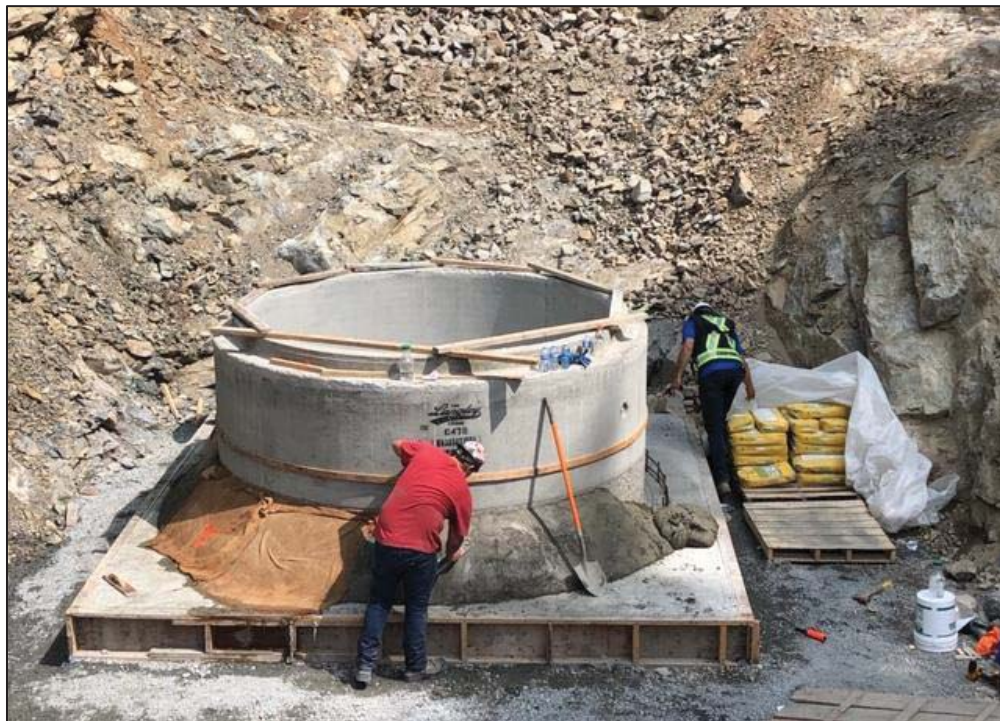
Figure 26–Residual Solids Conveyance Line- Placing and finishing non shrink grout around pump station 3 wet well.
