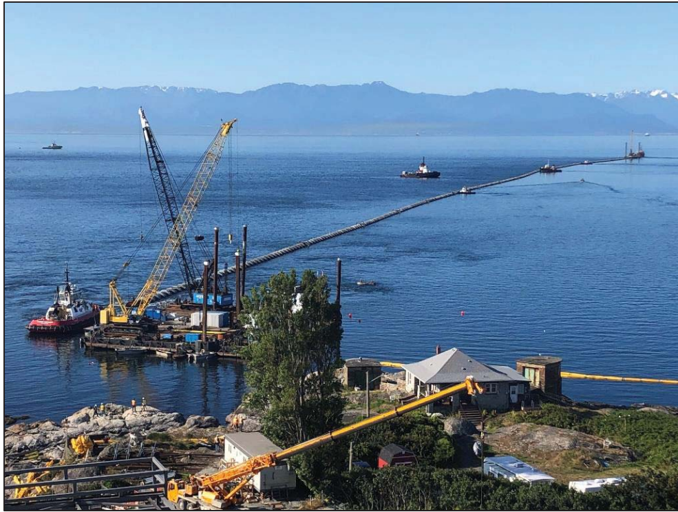
Figure 2– McLoughlin Point Wastewater Treatment Plant- Floating the marine outfall into place prior to submerging.
