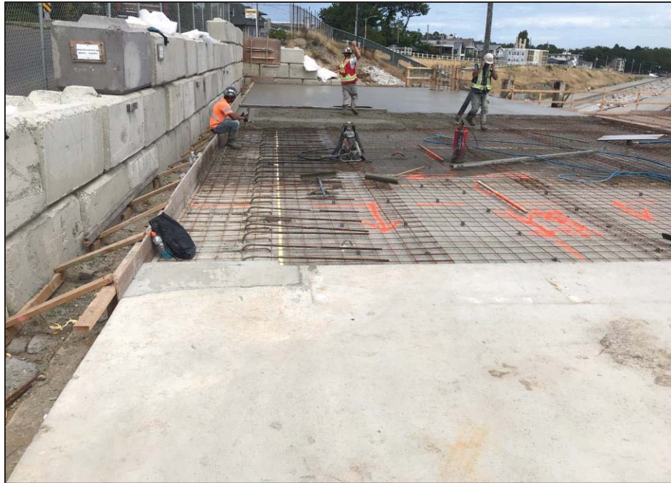
Figure 11–Clover Point Pump Station- Roof slab concrete pour.
