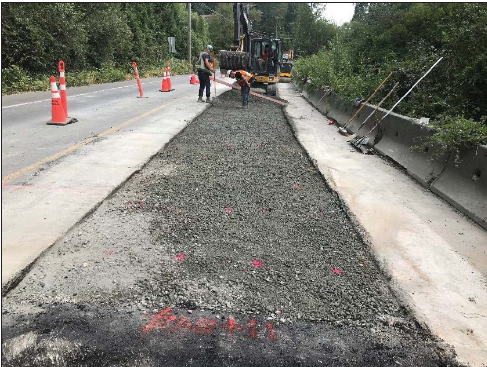
Figure 23–Residual Solids Conveyance Line- Prepping for base asphalt in segment 3 Interurban Road between Quayle Road and Goward Road.
