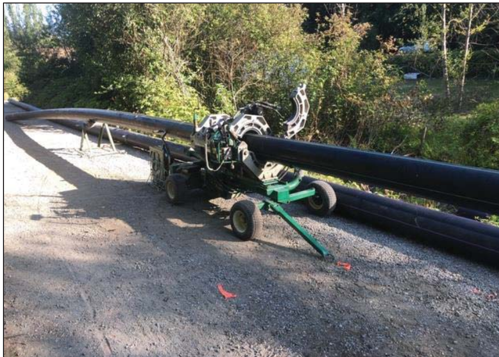
Figure 28–Residual Solids Conveyance Line- Setting up to fuse high density polyethylene pipe at pump station 2, Interurban Trail.
