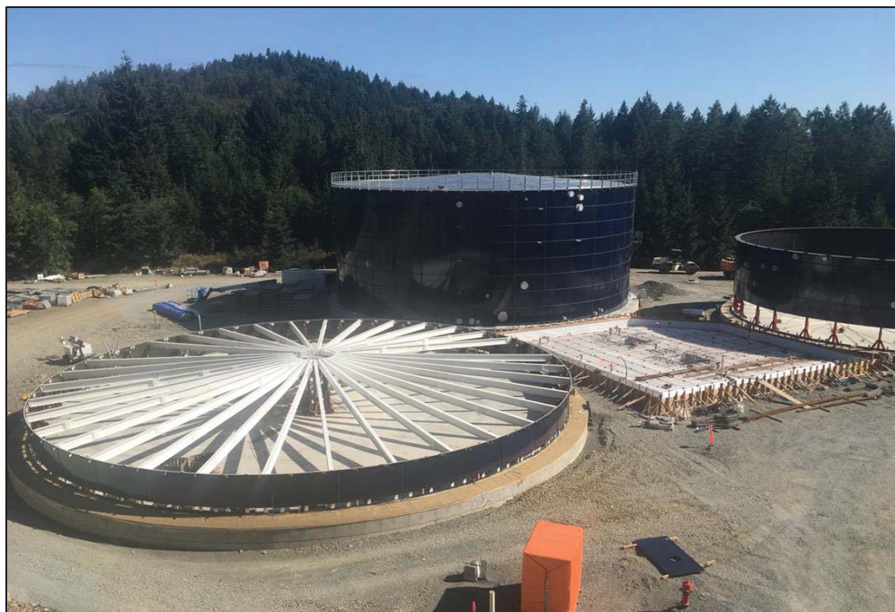
Figure 10– Residuals Treatment Facility- Site photo showing progress of Digester #2, Digester Equipment Building and Digested Solids Storage Tank.
