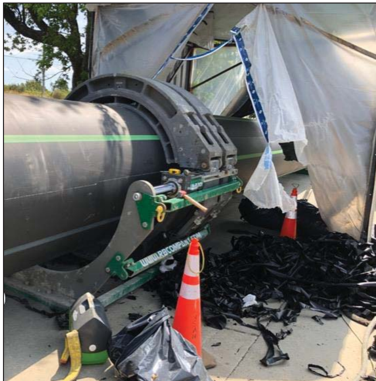
Figure 17–Macaulay Point Pump Station- Fusion welding sections of high density polyethylene pipe on Anson Street.
