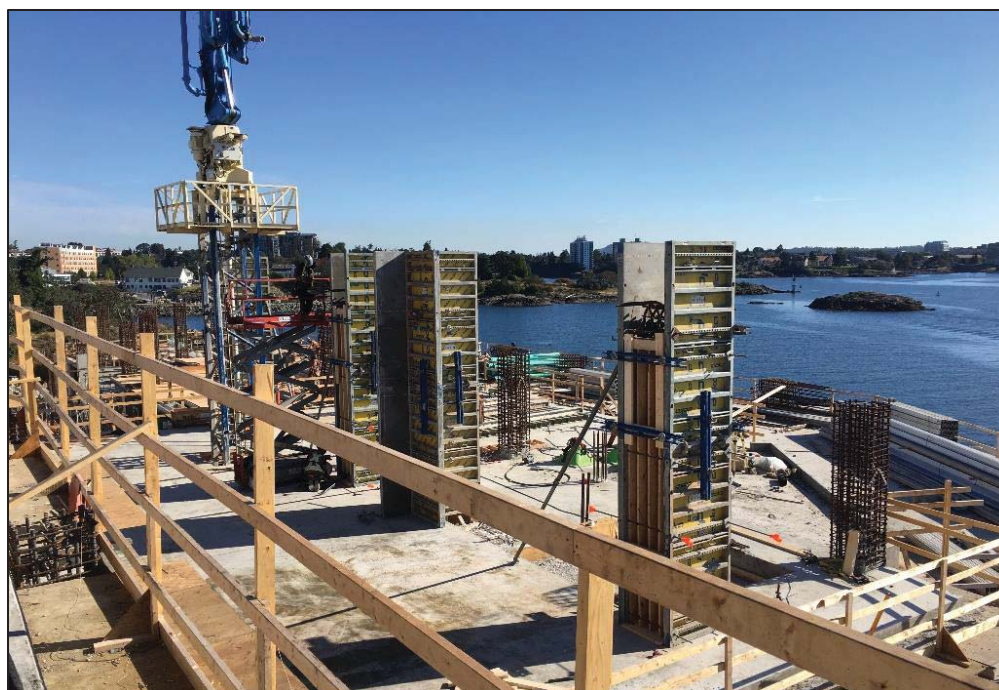
Figure 6– McLoughlin Point Wastewater Treatment Plant- Forming columns of the third level suspended slab.
