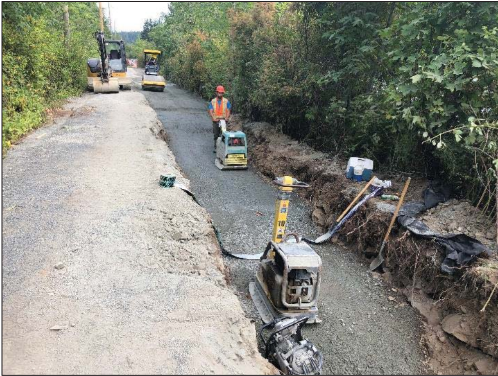
Figure 22–Residual Solids Conveyance Line- Backfilling and compaction at Interurban Trail segment 4 between Wallace Drive and Hartland Ave.
