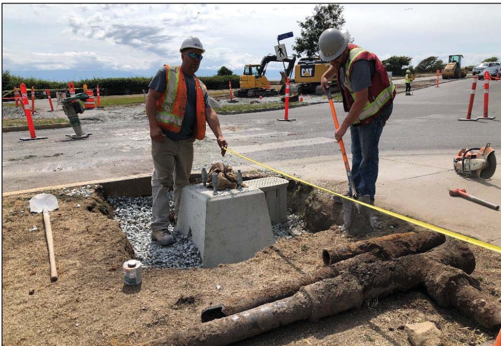
Figure 20–Clover Forcemain-- Streetlight Base and underground electrical ducting installed (Dallas at Cook St.).
