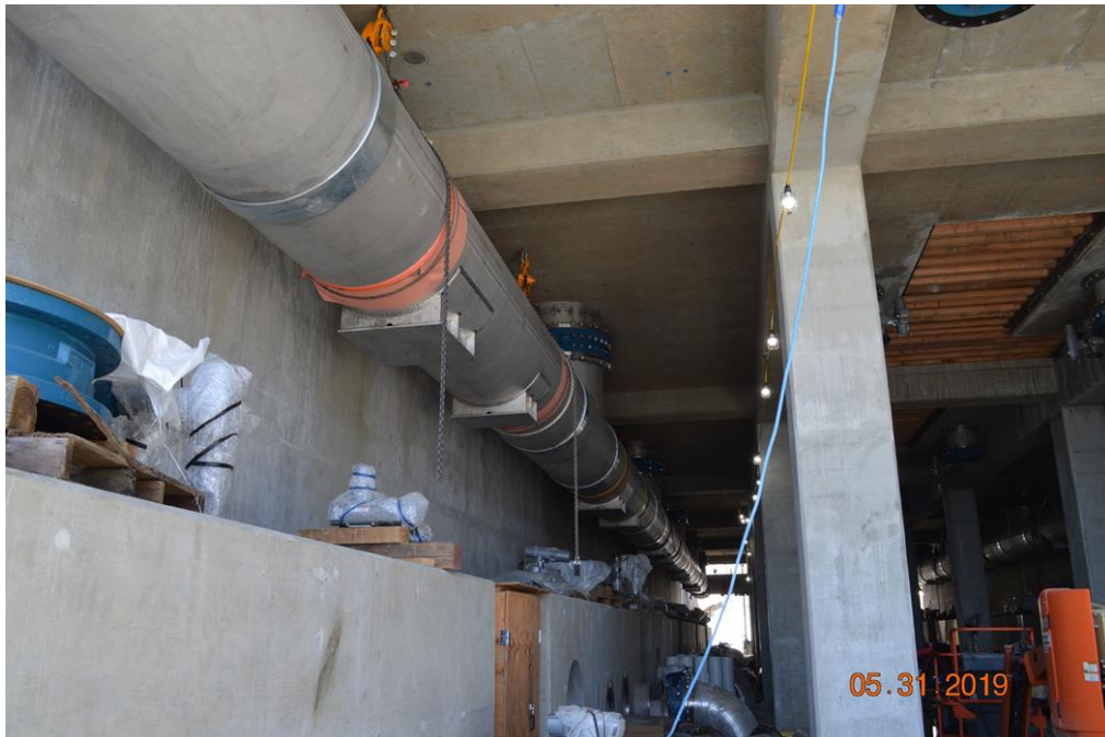
Figure 4 – Mcloughlin Point Wastewater Treatment Plant – 42" BWW header
