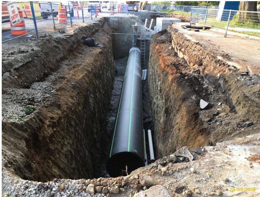
Figure 22 – Clover Forcemain: Installing forcemain towards Douglas Street.
