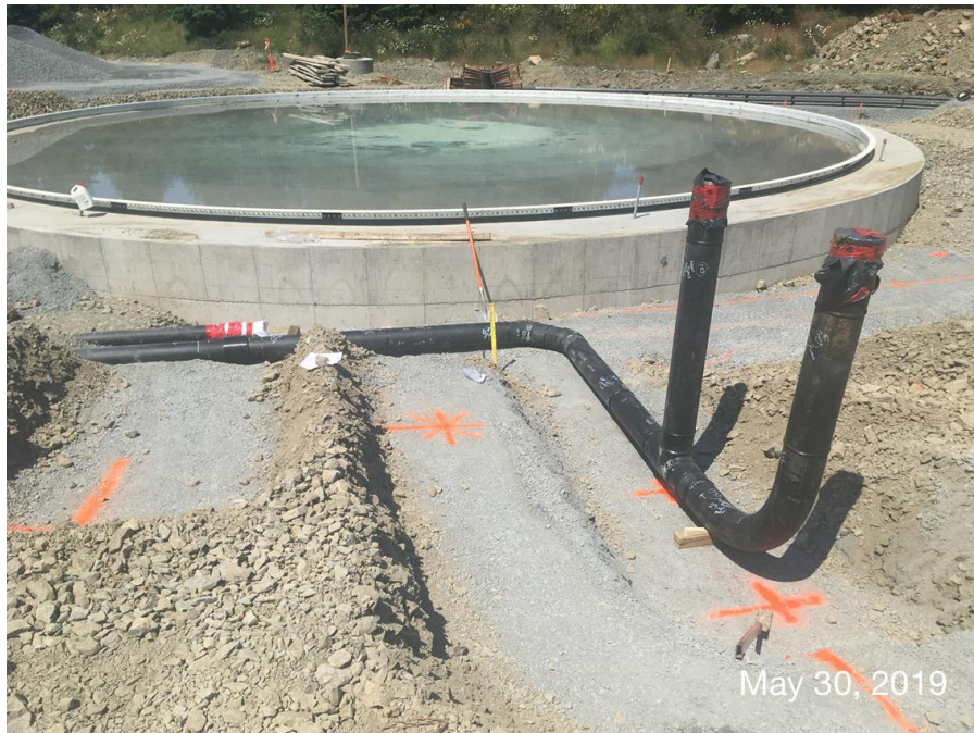
Figure 11– Residuals Treatment Facility – high density polyethylene process piping assembly installed at south side of residual solids.
