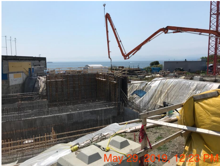
Figure 19 – Macaulay pump station & forcemain – pouring the second lift of the exterior wall SW corner.
