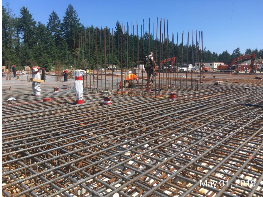
Figure 9– Residuals Treatment Facility – installation of reinforcing steel for Residuals Handling Building slab..
