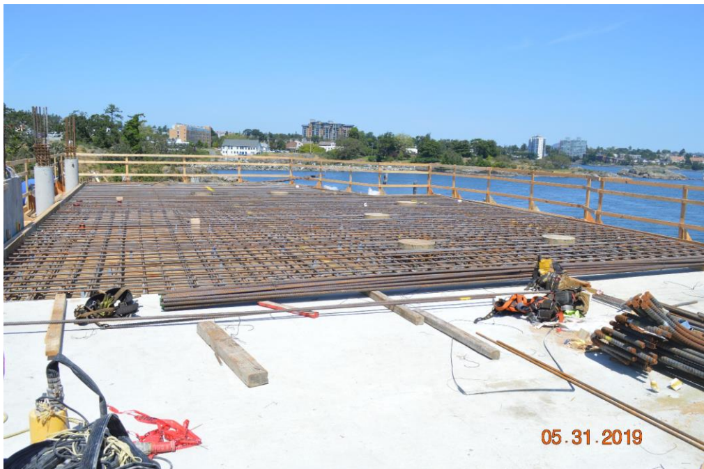
Figure 3 - Mcloughlin Point Wastewater Treatment Plant – Rebar completed for Operations & Maintenance building level 2 suspended slab pour
