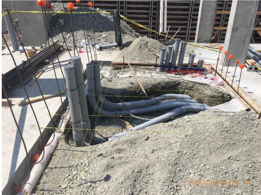
Figure 7 – Mcloughlin Point Wastewater Treatment Plant – installing conduit for Operations & Maintenance building electrical room.
