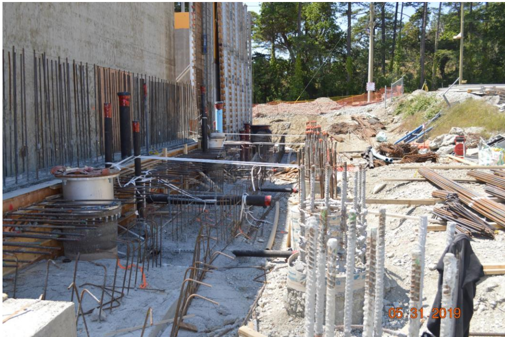
Figure 2 – Mcloughlin Point Wastewater Treatment Plant – Phase 3 piling completed at pump room at north end of Lamella plate settlers.
