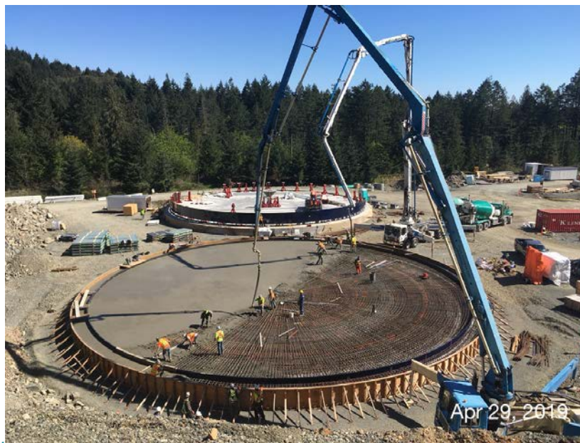
Figure 11 – Residuals Treatment Facility: concrete being placed in digester #2 floor slab and erection of bolted steel tank wall in the background.
