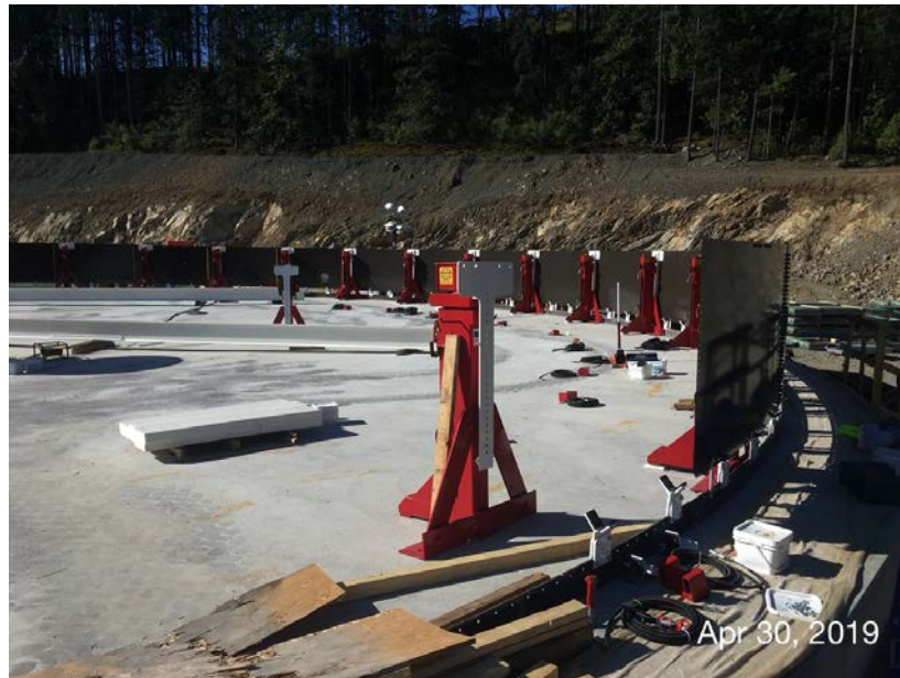
Figure 10 – Residuals Treatment Facility: assembly of first ring of bolted steel tank in Digester #1.
