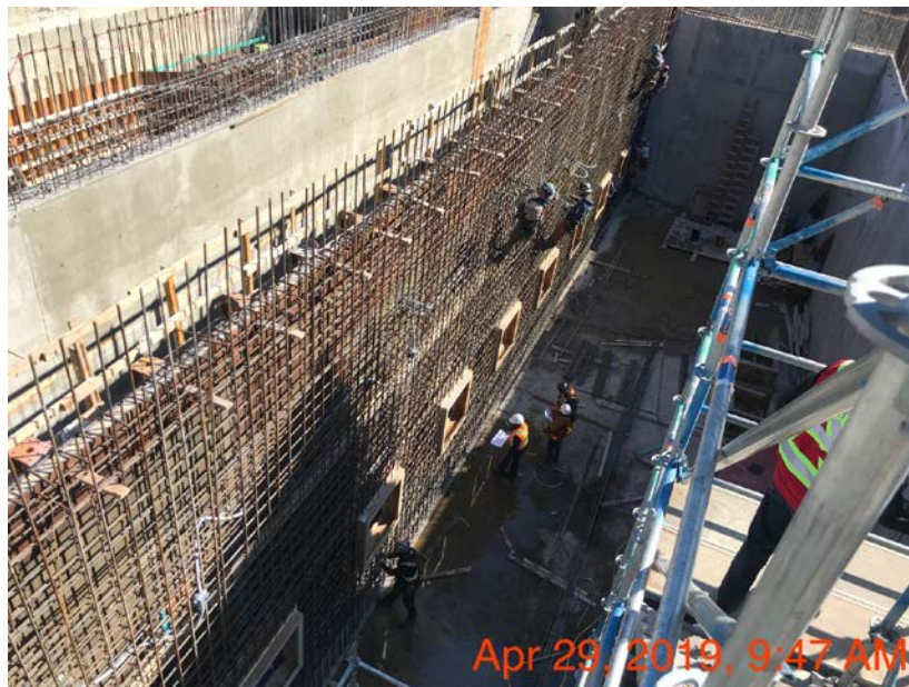
Figure 19 – Macaulay Point Pump Station: installing rebar, electrical conduits and formwork for interior wall along gridline C.
