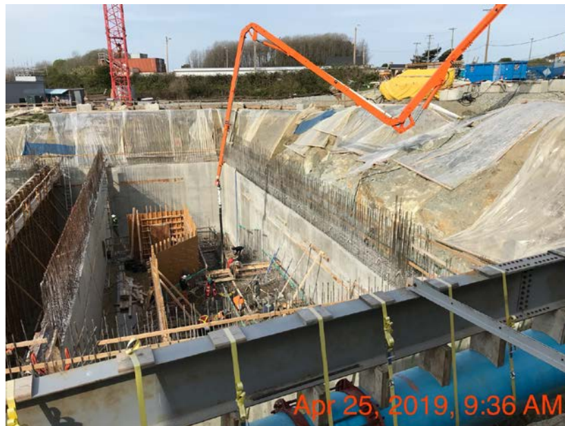
Figure 20 – Macaulay Point Pump Station: concrete pour of the topping slab in the inlet channel.
