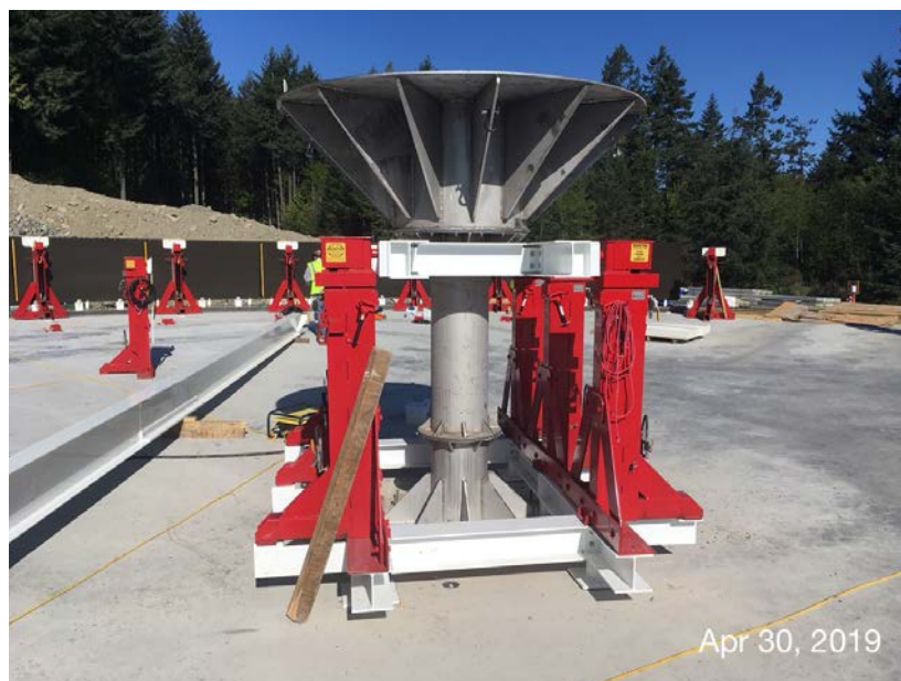
Figure 9 – Residuals Treatment Facility: hydraulic jacks set up around central roof support column.
