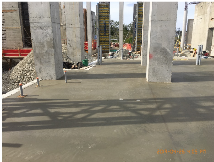
Figure 8 – McLoughlin Point Wastewater Treatment Plant: pouring slab.
