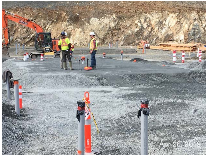
Figure 12 – Residuals Treatment Facility: placing, grading, compaction and shaping of base gravels beneath Residuals Handling Building.
