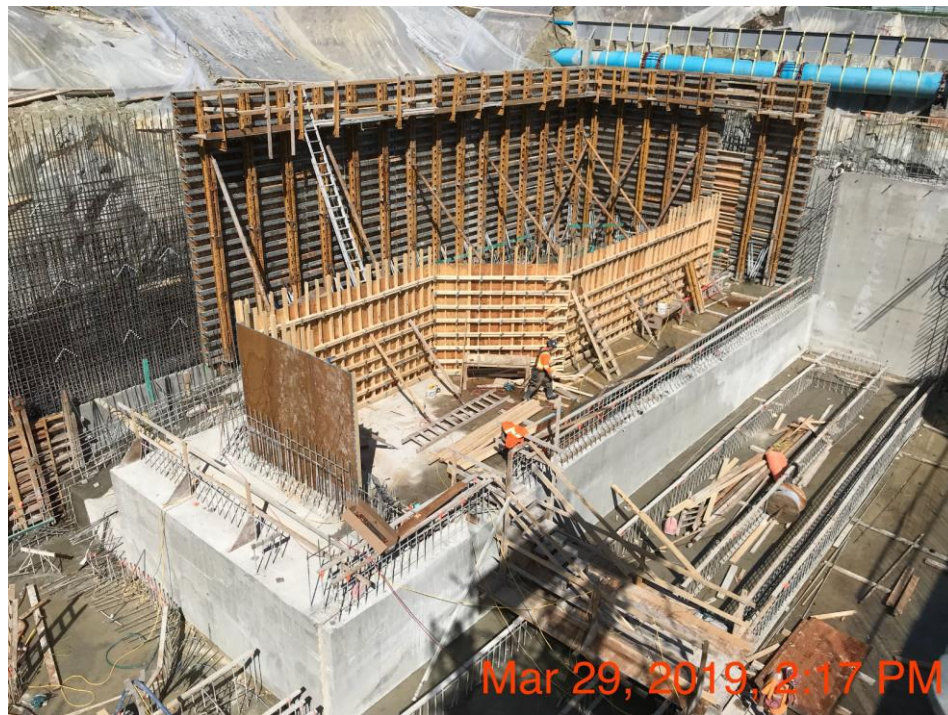
Figure 14 – Macaulay Point Pump Station: Installing rebar for the exterior wall pour and installing interior and exterior formwork.
