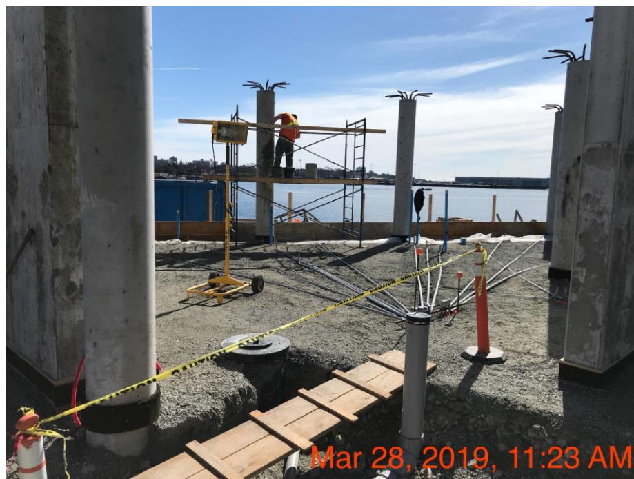
Figure 4 - McLoughlin Point Wastewater Treatment Plant: installation of electrical conduit in Lab area.
