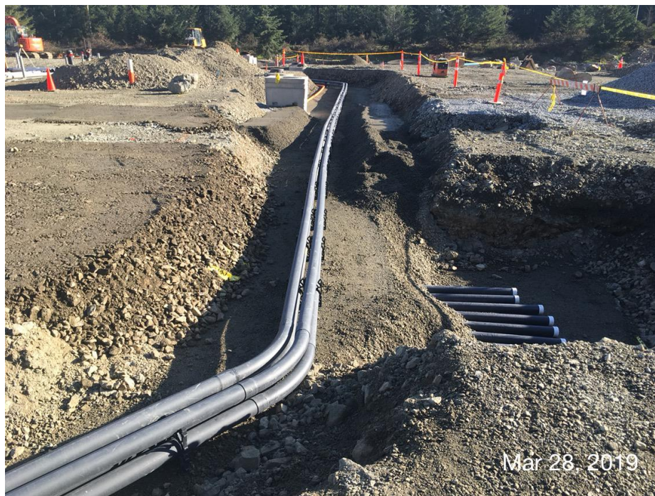
Figure 10 – Residuals Treatment Facility: installation of hydro and communications conduits east side of future centrifuge building.
