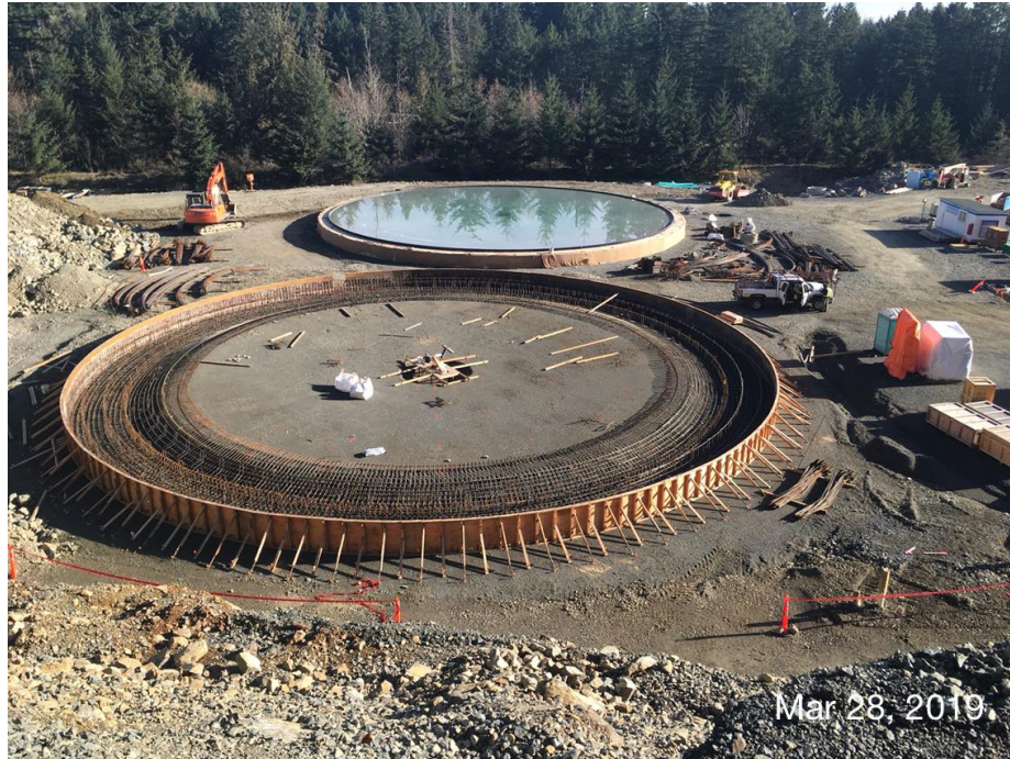
Figure 9 – Residuals Treatment Facility: digester #1 flooded for curing, and installation of reinforcing steel for first pour on digester #2
