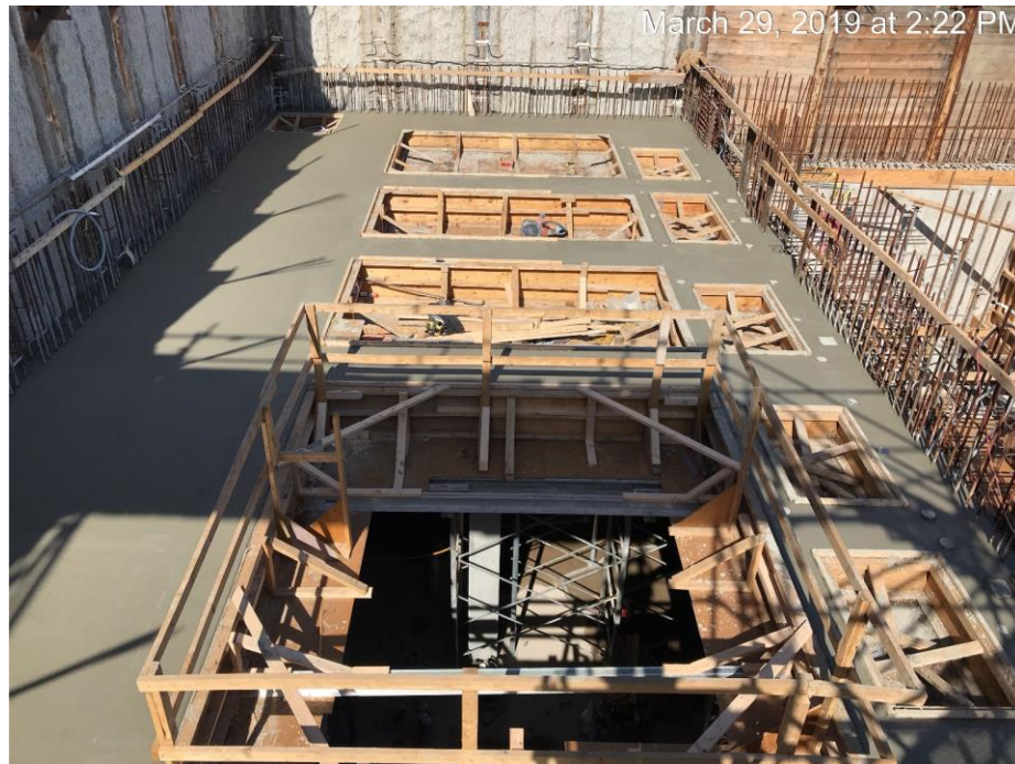
Figure 11 – Clover Point Pump Station: Overview of suspended slab 02 after concrete was poured.
