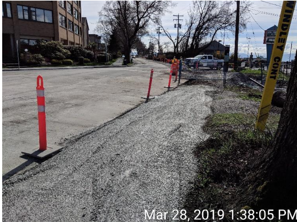
Figure 19 – Clover Forcemain: Dallas Road – Road restoration at St Lawrence and Dallas Rd..
