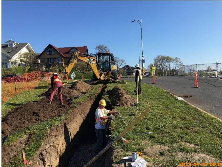
Figure 9 – BC Hydro contractor excavating for duct bank and pull box west side of Clover Point Road.
