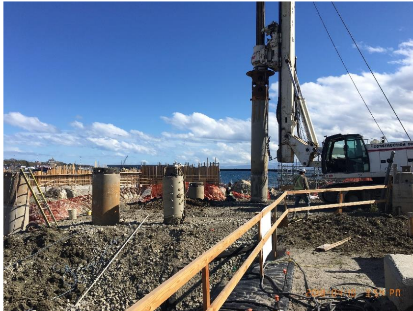
Figure 4 – Drilling piles in the BAF area
