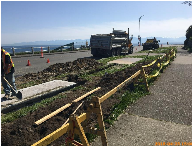
Figure 10 – BC Hydro contractor installing duct bank and pull box on north side of Dallas Road
