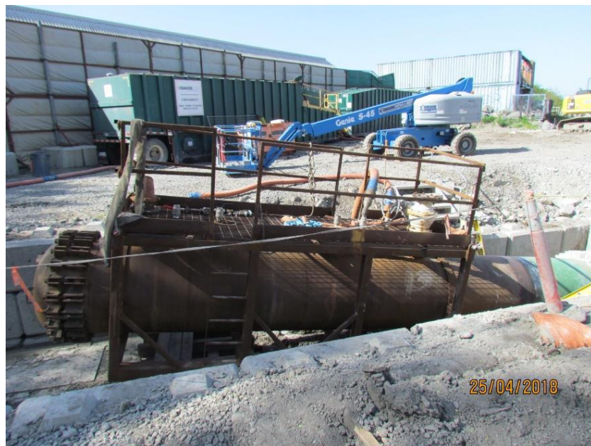
Figure 7 – Hydrostatic test head installed on the Ogden end of the Harbour Crossing pipe.
