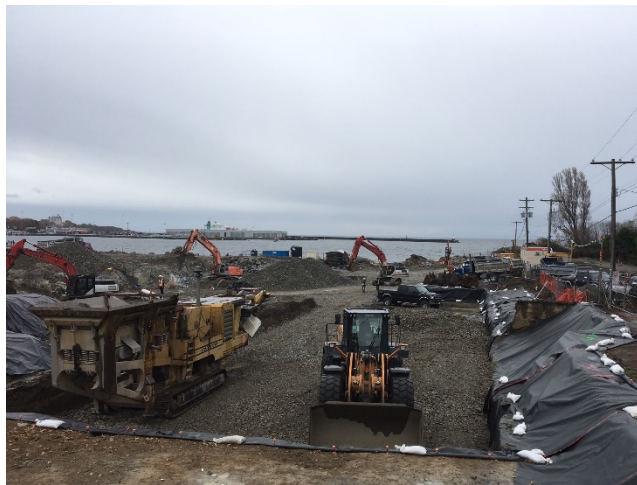
Figure 6 – Slope stabilization and protection
