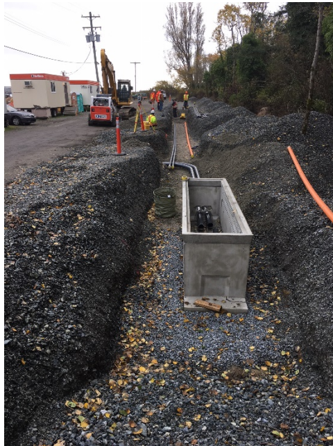
Figure 5 – Installation of BC Hydro ductbank
