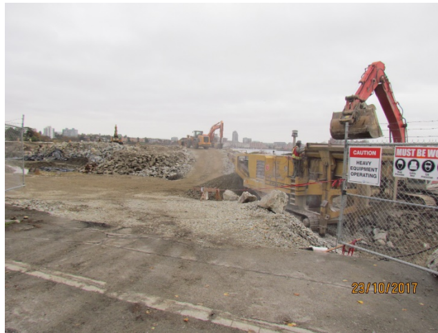
Figure 2 — Crushing of blast rock
