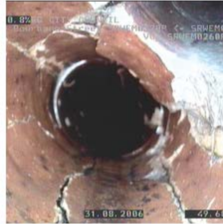
DETERIORATING SEWER PIPE
