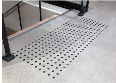
Example of dark stud-style TWSIs that provide both contrast and tactile information.
