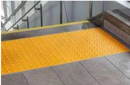
Photo demonstrates the correct placement of TWSIs at the tops of stairs.
