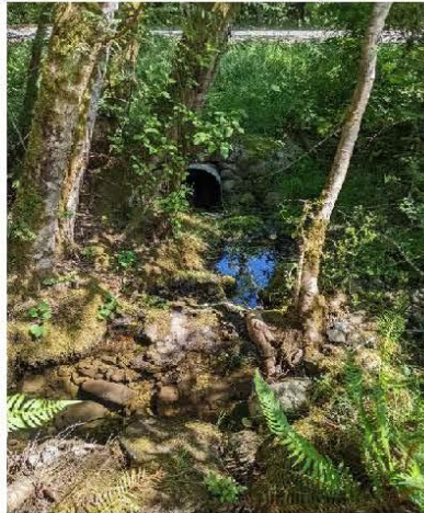
Photo 4. North (downstream) view of watercourse and culvert under Brecon Drive June 30, 2022.
