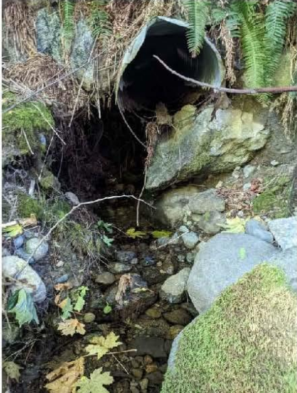
Photo 9. South (upstream) view of dilapidated culvert on north side of Brecon Road. June 30, 2022.
