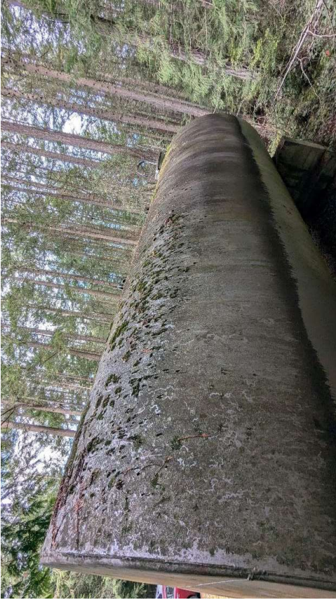
Figure B-6 Exterior Top of Tank
