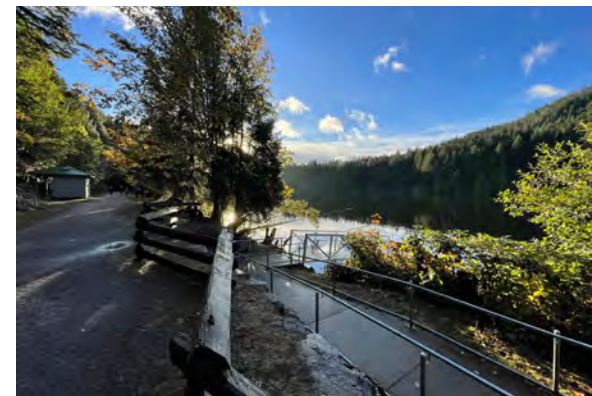
RAMP AND DOCK
