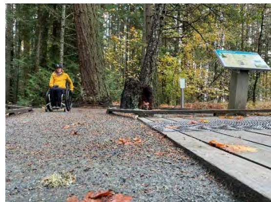
Figure 13 Packed Crushed Aggregate with Fines Provides for an Accessible Trail Surface with Minimal Tread Obstructions
