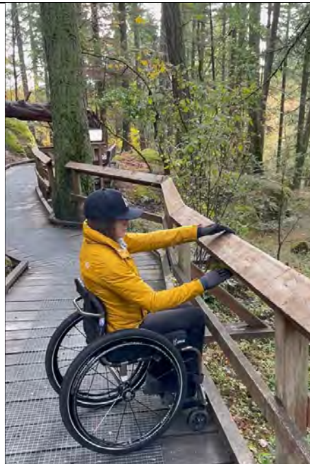
Installation Height & Dimensions of Railings Can Block Views Along Trails
