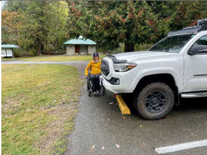
Wheel Stop Location Allows Vehicles to Block Narrow Path from Parking Lot to Trail
