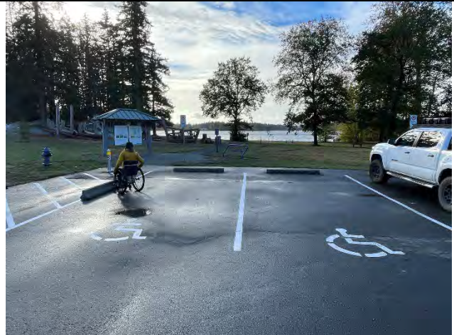
Accessible Stalls Do Not Provide Space for Vans with Side Loading Devices
