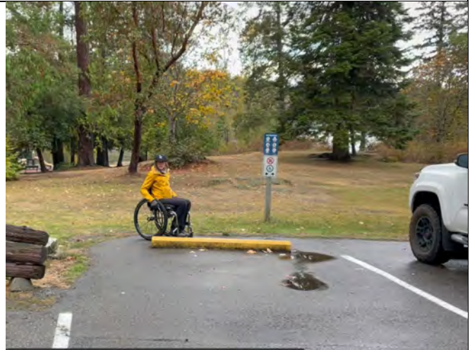
Access from Accessible Parking Stall to Park's Trail System is Blocked by Parking Stall
