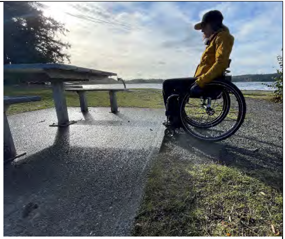
Accessible Picnic Table Provides for Choice but Transition and Adjacent Surfacing Limits Access
