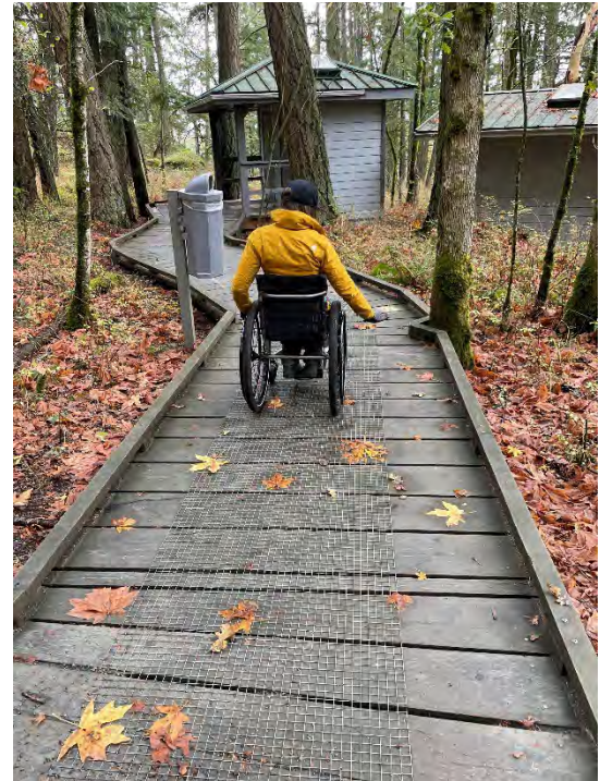
Figure 12 Wire Grid Installed on Boardwalk Improves Traction, Limits Vibrations for People with Mobility Devices and reduces maintenance requirements, Guide Rail Provides Tactile Orientation for People with Visual Impairments and Limits Potential for Mobility Devices to Leave the Tread
