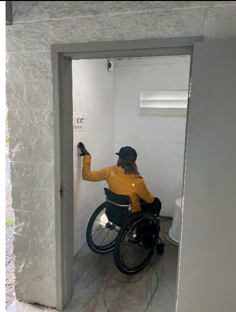
Height & Placement of Grab Bars, Coat Hooks, Inside Door Handles, Toilet Paper Dispensers and Hand Sanitizer Can Greatly Impact Functionality of the Toilet Building for People with Disabilities
