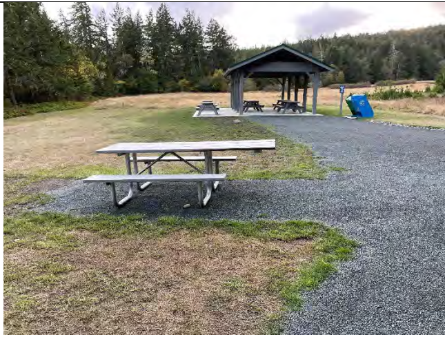
Surfacing Around Picnic Table Limits Ability to Travel Around Table & Accessibility Overhang on One End Limits Visitor Choice
