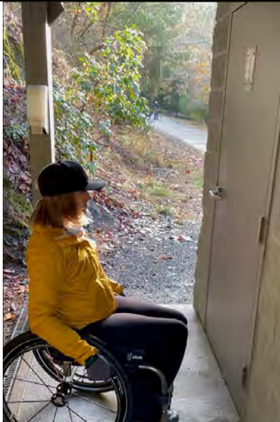
Direction of the Door Swing Makes it Very Difficult to Access the Toilet from the Concrete Platform
