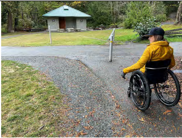
Unsuitable Trail Tread Widths and Transition from Pavement to Gravel
