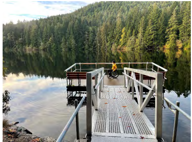
Figure 3 Accessible Fishing Pier at Durrance Lake Mount Work Regional Park
