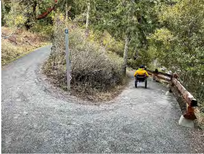
Overly Steep Trail Grades Limit Access to the Beach Which is the Most Desired Destination
