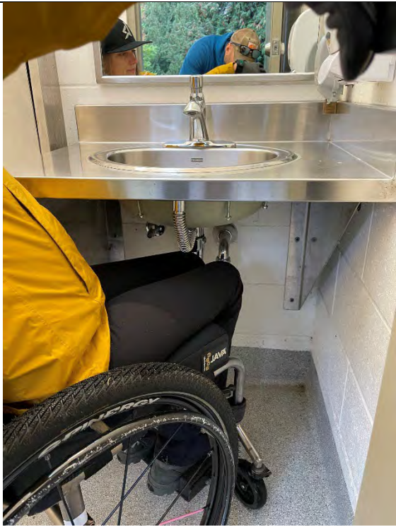
Limited Access to Approach Sink
