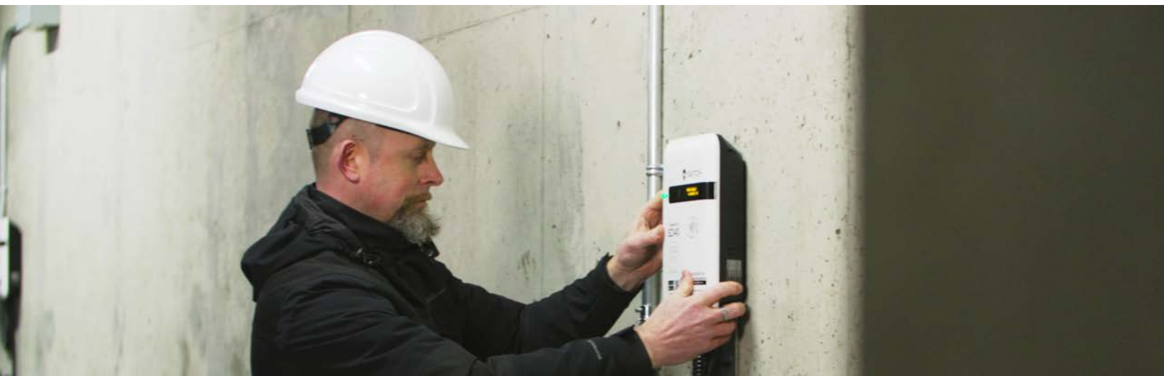
Electrician installing an EV charger
