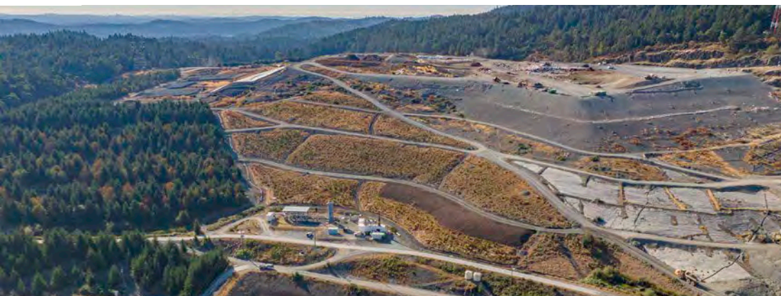
Hartland Landfill and the Landfill Gas Plant
