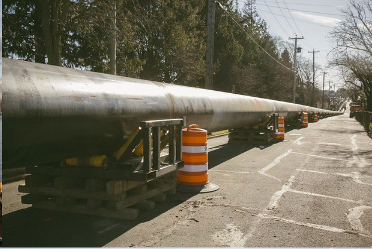
92 km Conveyance System
