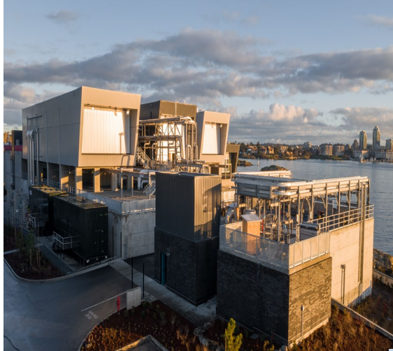
McLoughlin Treatment Plant
