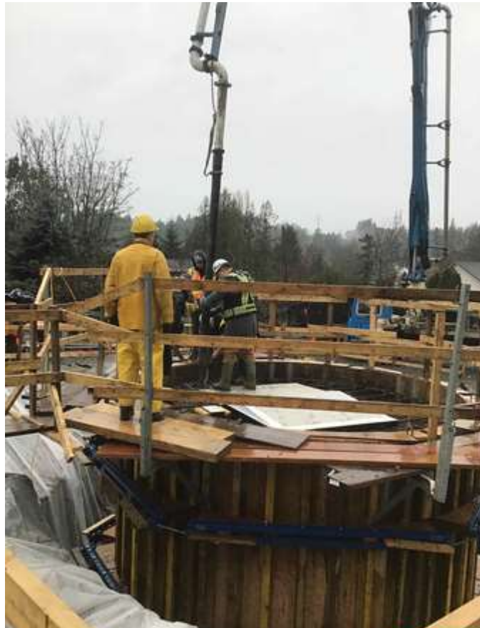
Figure 26 –Residual Solids Pump Stations - Pump Station 1- Wet well concrete pour in progress.
