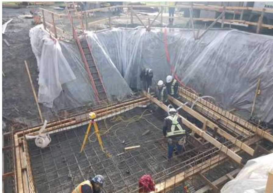
Figure 27–Residual Solids Pump Stations – Installing formwork and reinforcing steel for Marigold pump station valve chamber.
