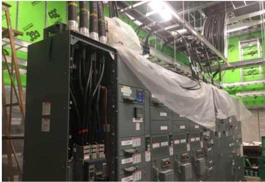
Figure 7– Residuals Treatment Facility- Residuals Handling building electrical room motor control centres.
