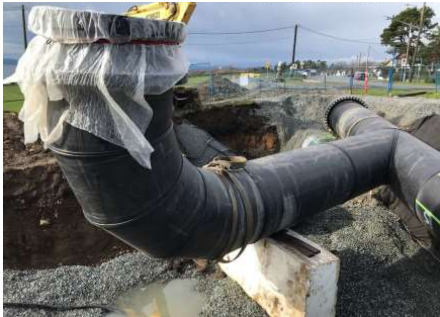
Figure 13–Clover Point Pump Station- Forcemain blind flange is installed and pigging station pipe bedding is being placed.
