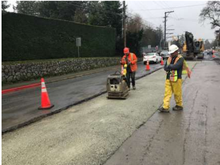
Figure 24-Residual Solids Pipes - Compaction being completed on prep work for temporary paving on Interurban Road.
