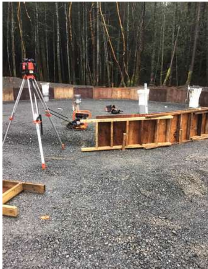
Figure 25–Residual Solids Pump Stations– Hartland Water System Improvements – Installation of formwork for the reservoir slab.
