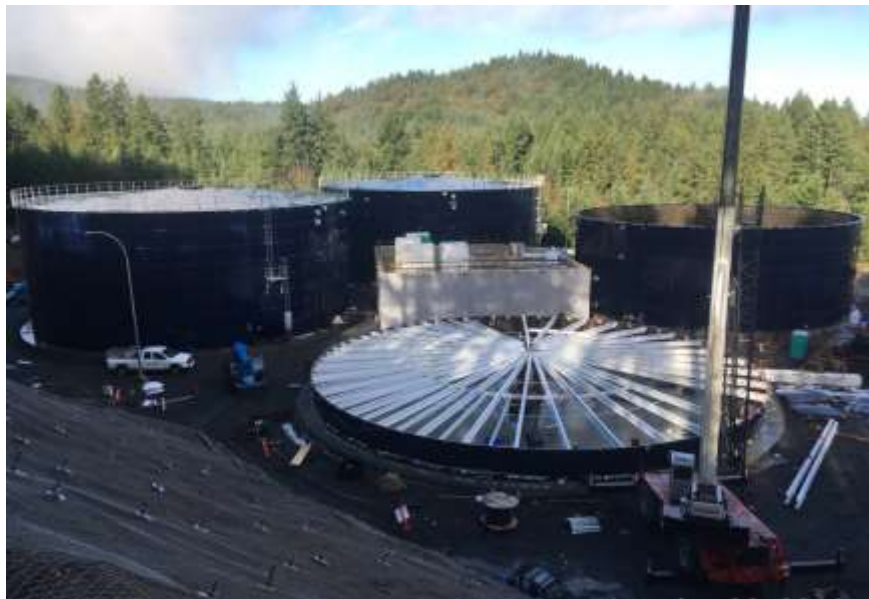
Figure 8– Residuals Treatment Facility- Digester 3 construction in progress.
