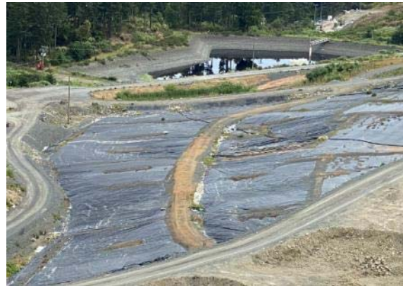
Photo 4.2 - Temporary Woven Liner (Area S10, S11)
