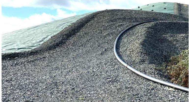
Photos 4.8a & 4.8d - Emission Hotspots, Edge of Geomembrane Liner and Damaged Liner (Area S1)
