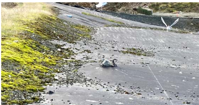
Photos 4.9a & 4.9b - Temporary Liner Puncture (Area S10)
