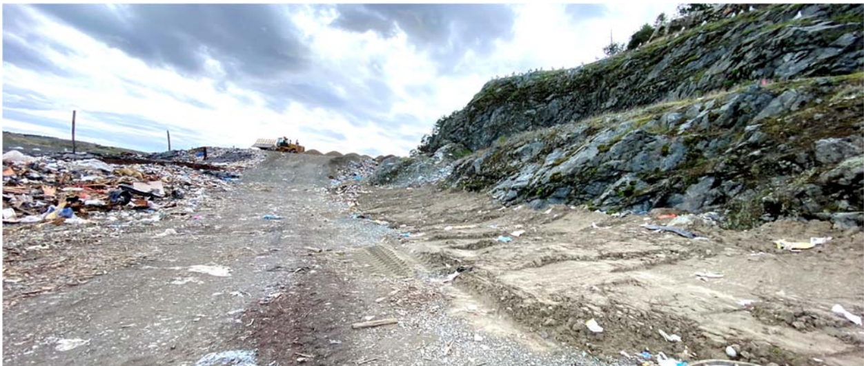
Photo 4.5 - Rock Wall Drainage Blanket Clay Plug, October 2020
