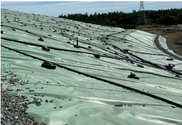
Photo 4.3 - Textured Geomembrane (Area S1)
