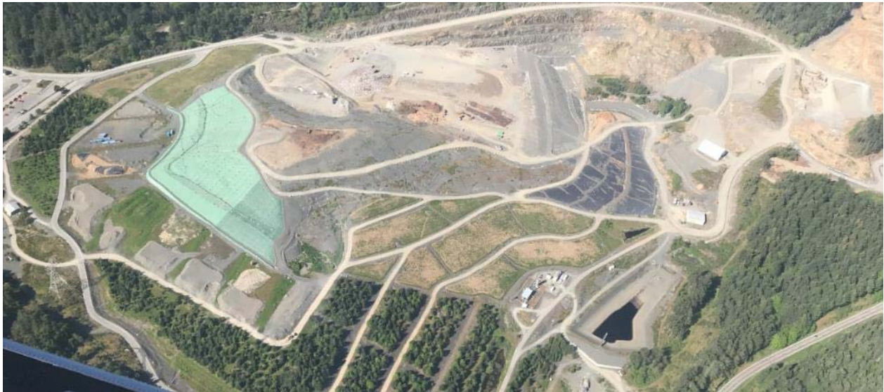
Photo 1.1 - Hartland Landfill Aerial Photo
