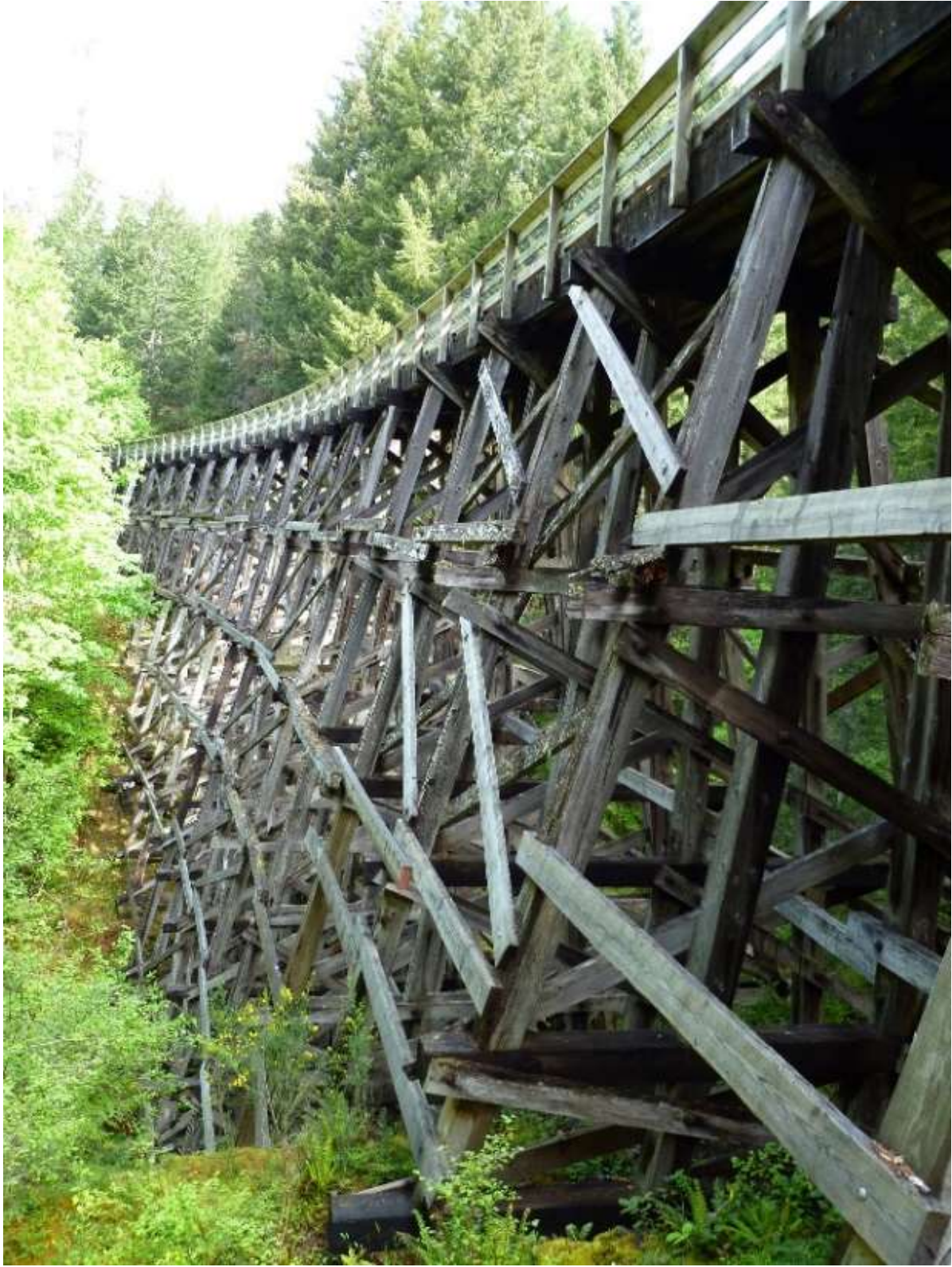
Todd Creek Trestle – Looking North
