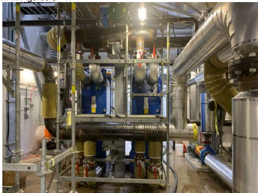
Figure 6- Residuals Treatment Facility- Pipe insulation being installed on Dryer building process piping.
