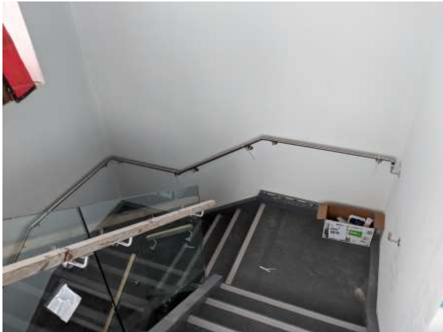
Figure 5– McLoughlin Point Wastewater Treatment Plant- Handrail installed in Operations & Maintenance main entrance stairwell.
