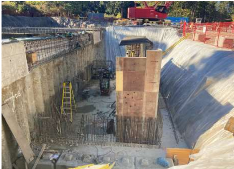
Figure 18–Arbutus Attenuation Tank- Valve chamber wall formwork installed.
