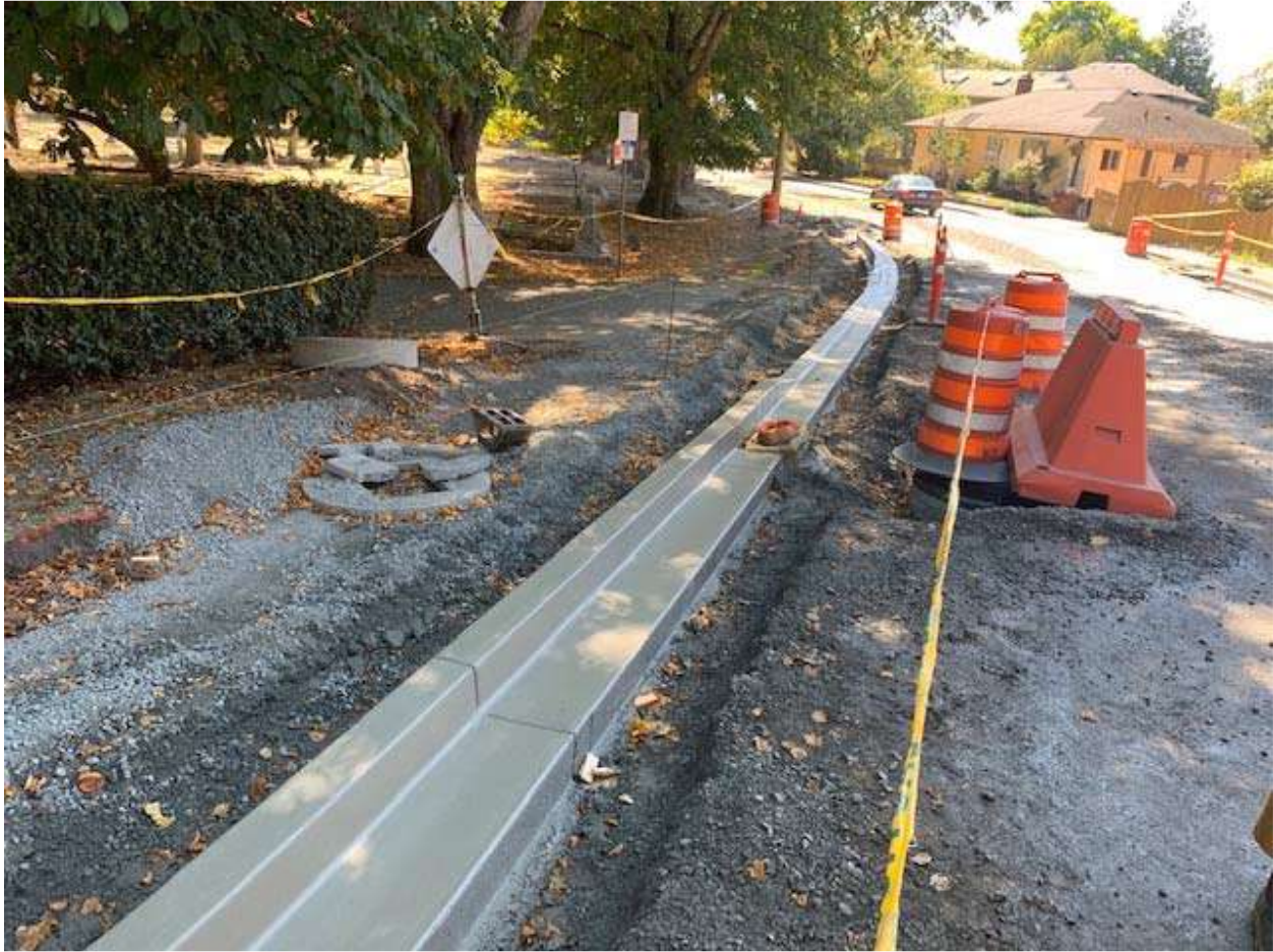
Figure 20–Trent Forcemain- Curb work completed on Memorial Crescent.
