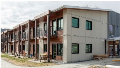
132 Corbett Rd. Phase II Opened 2020
