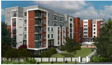
RHFP/BC Builds - Campus View 2027
