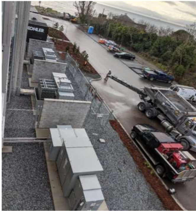
Figure 3 – McLoughlin Point Wastewater Treatment Plant- Gravel installation along the generator area.
