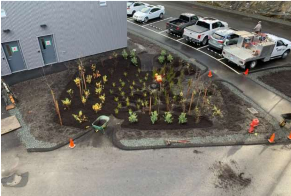
Figure 5 – Residuals Treatment Facility- Landscaping installation.
