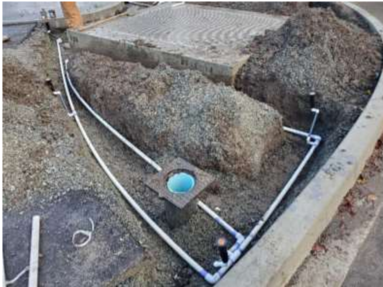
Figure 10 – Residual Solids Pump Stations–Pump Station 2 – Installation of irrigation and sprinkler heads.
