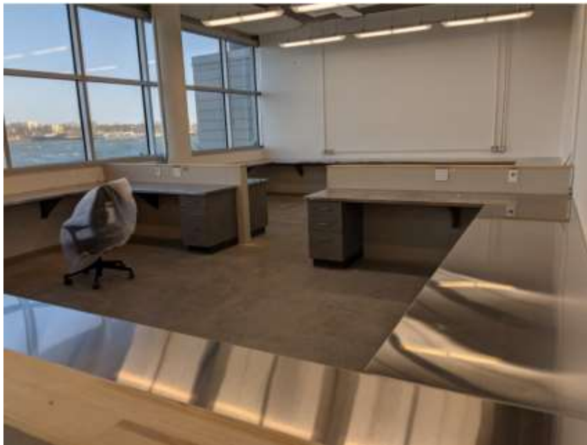
Figure 2 – McLoughlin Point Wastewater Treatment Plant – Aluminium countertops and electrical outlets installed in instrumentation workshop
